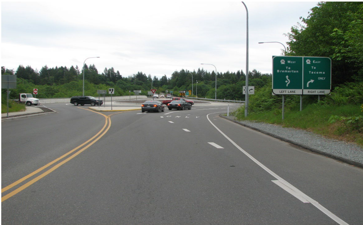
Figure 8. Site 2: Borgen Boulevard in Gig Harbor, Washington (Street View)
