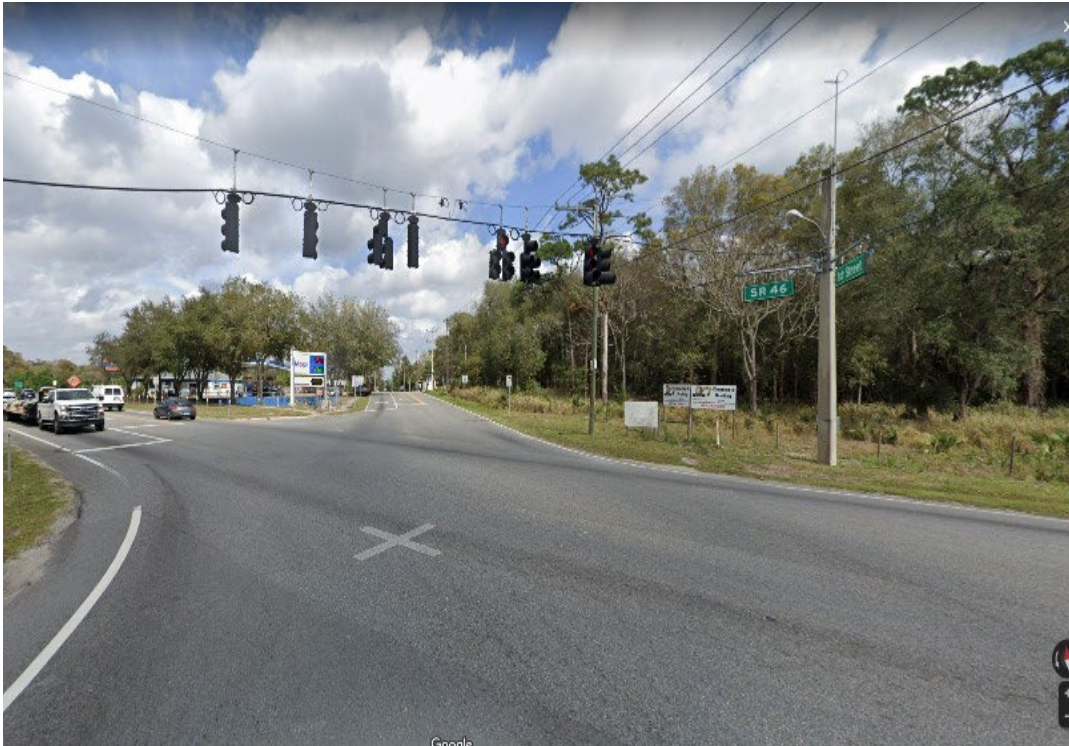
Figure 20. Site 4: FL-46 and CR-426 (CR-426, Northbound Direction)
