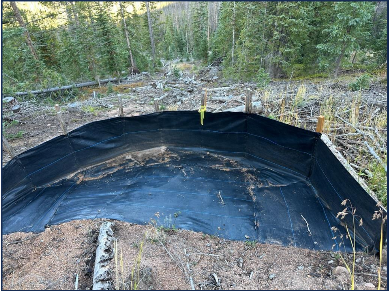
Figure 2. Photo of a sediment fence on a bare tether road. The tether road transitions to slash cover downslope of the fence. The fence dimensions are approximately 4 m wide (i.e. the 4 m width of the tether road), 1.5 m deep, and 0.5 m high.
