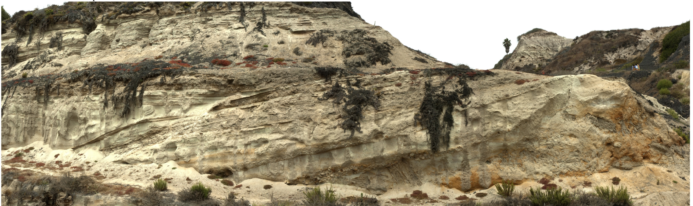
Channel 3.4 Bank Collapse
