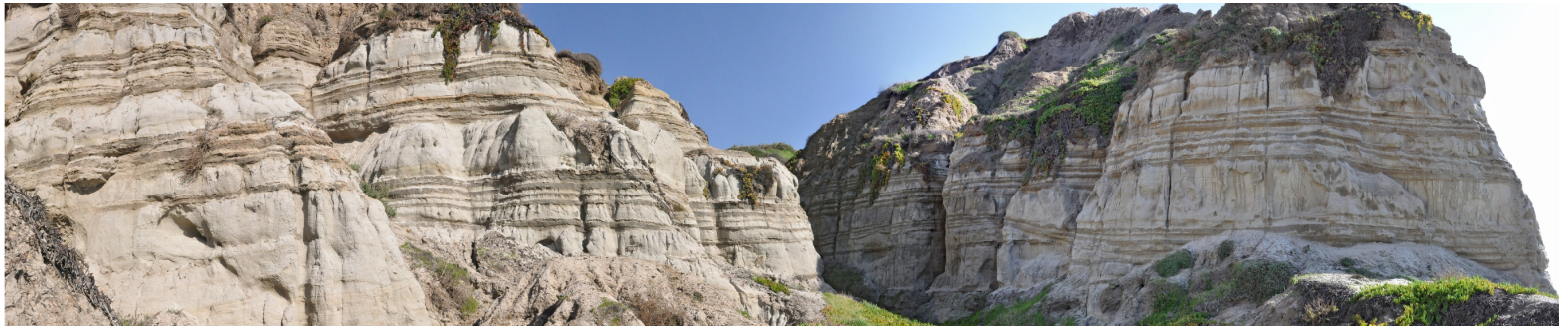
North Gulley - South Wall
