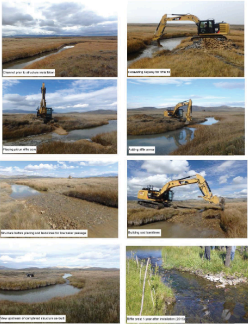
LONG CREEK, CENTENNIAL VALLEY, MT INCISED CHANNEL RESTORATION PILOT PROJECT: Demonstration of Hardened Riffle Construction J-Bar-L Ranch 2014
