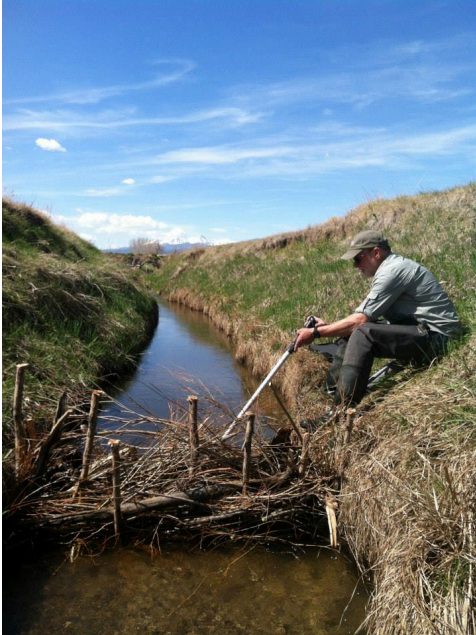
LONG CREEK, CENTENNIAL VALLEY, MT INCISED CHANNEL RESTORATION PILOT PROJECT: Demonstration of Hardened Riffle Construction J-Bar-L Ranch 2014
