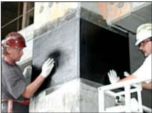
Figure 20: Column Strengthening [33]
