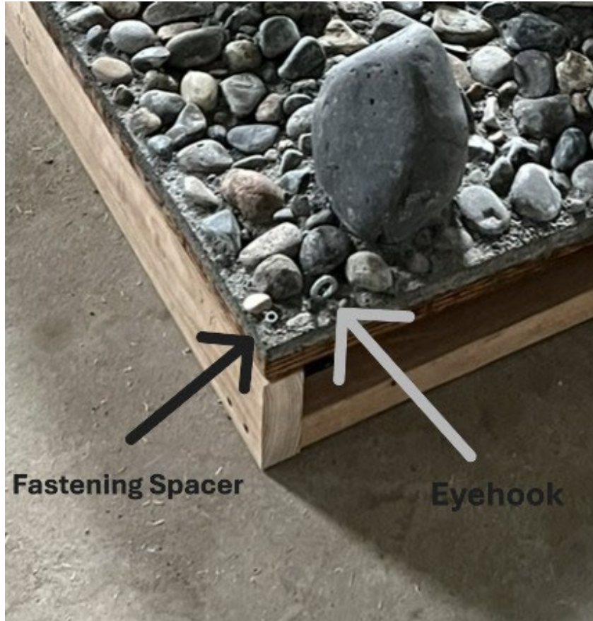
Figure 2: Corner of finished ramp panel showing fastening spacer and eyehook.
