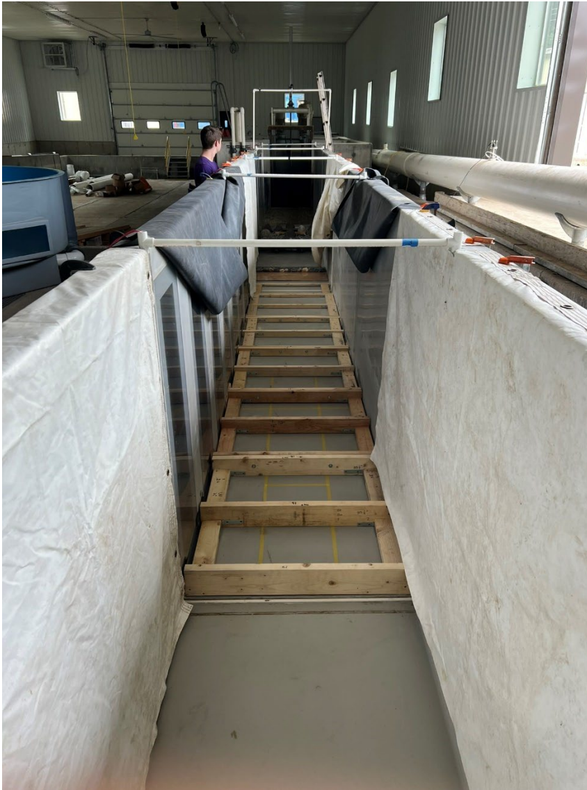
Figure 6: Ramp frame installed in flume looking downstream.
