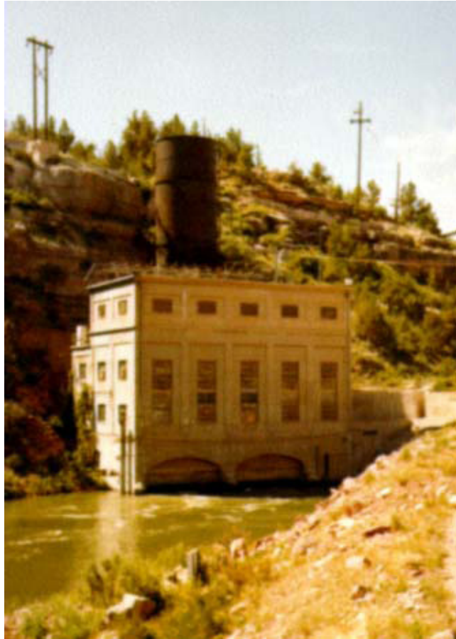
fig. 7 Guernsey Power Plant
