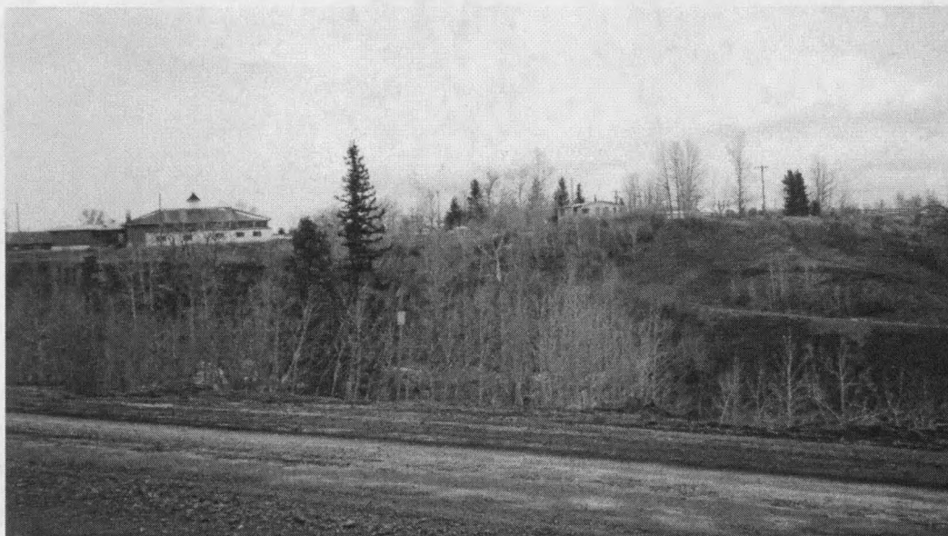
Figure 15. Wagon Road Westbound
