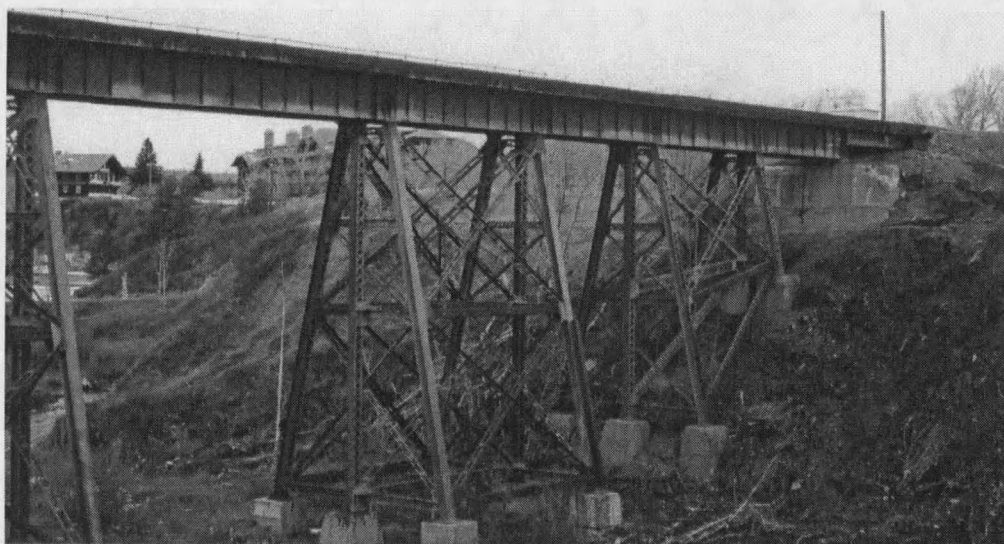
Figure 14. Original Road Connecting the Clarke and Dawson Townsites
