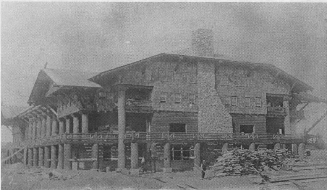
The construction of the Glacier Park Hotel in 1912. [Photographer unknown, Courtesy of GNP Archives (circa 1911-1912).]
