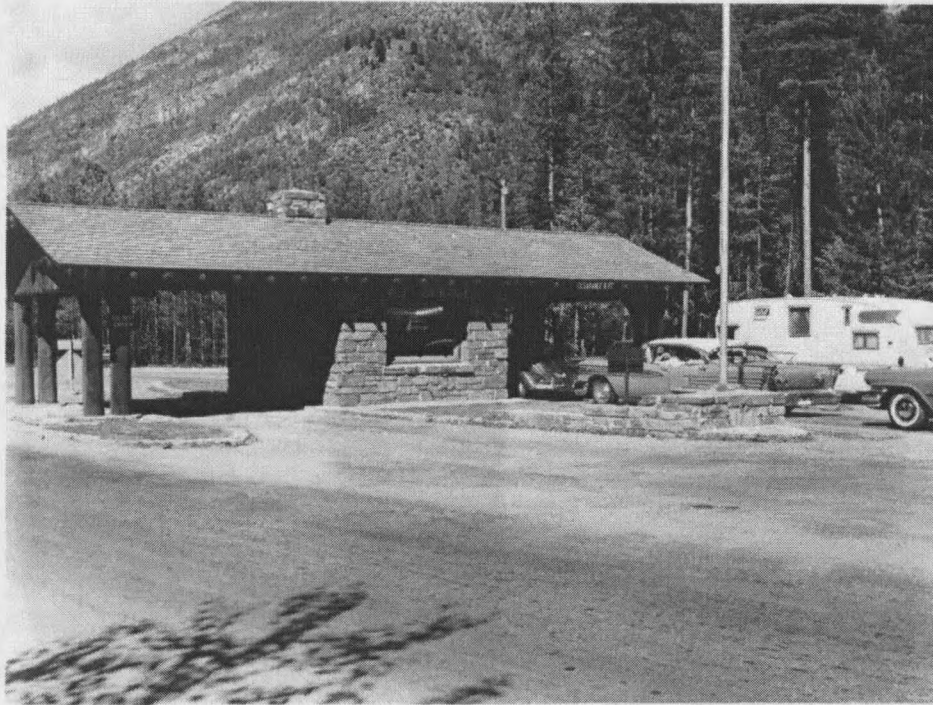
Figure 50. West Glacier Entrance Station
