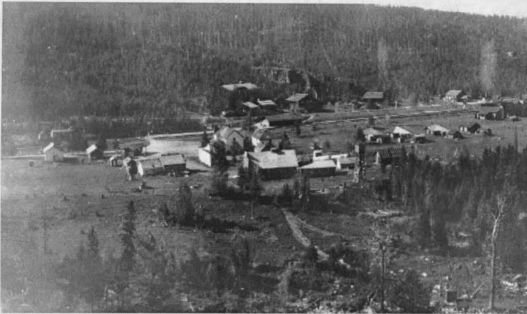
Figure 47. Aerial View of Belton in 1929
