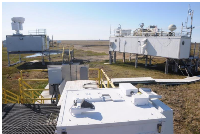
Figure 3-1. The ICI3 instrument (foreground) during its deployment at the ARM NSA site in Barrow, AK. Many of the other support instruments located at the ARM site are also shown in the image. (photo by Joe Shaw).
