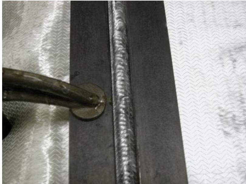
Figure 40: Fabric over polyethylene tubing constrained by steel bars.
