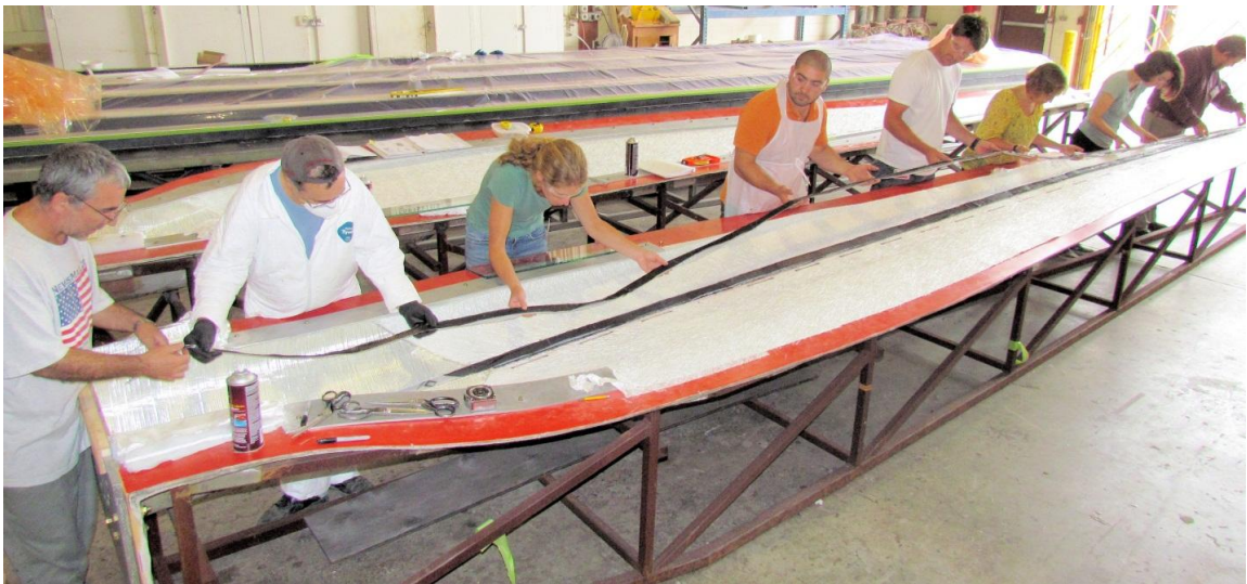
Figure 94: Photo showing a group effort to align the IP waves in the carbon spar cap.
