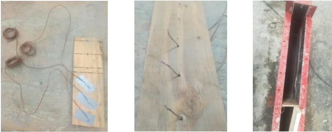
Figure 45. Formwork setup of the trial beam, showing thermocouple locations.
