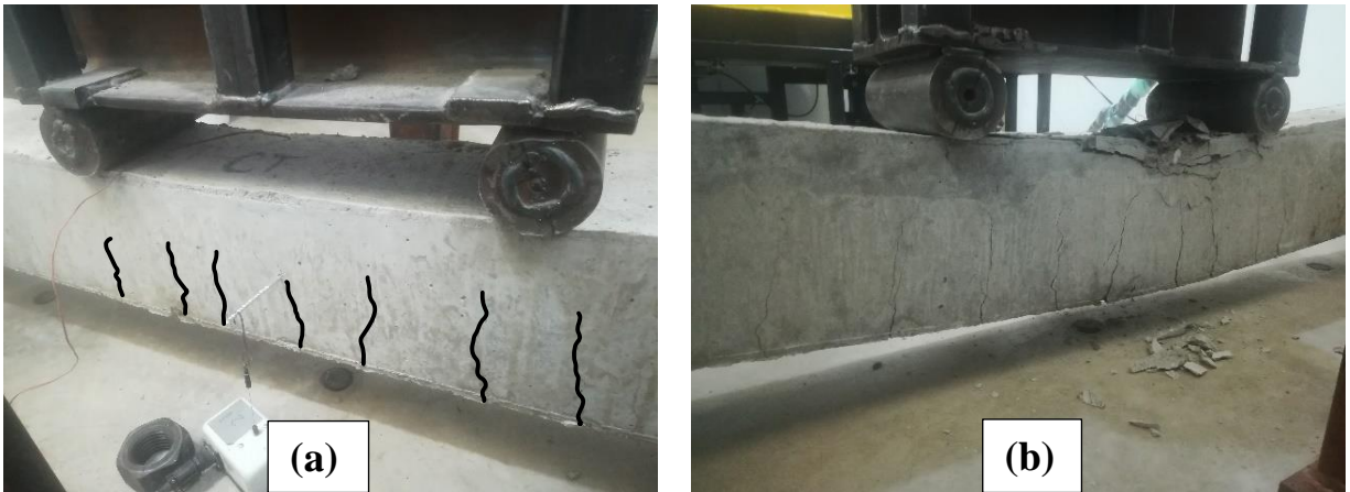
Figure 30. CBCT beam failure; (a) Flexural cracks forming throughout testing, (b) Concrete crushing at end of testing.
