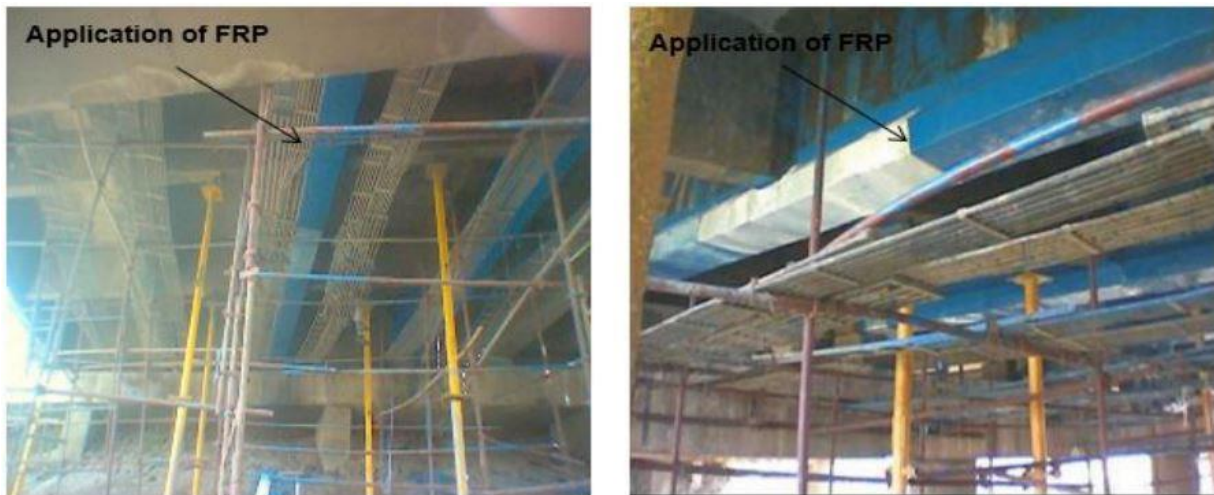
Figure 4. FRP application in Chaltan bridge, India (Abbas and Shahadat 2015).
