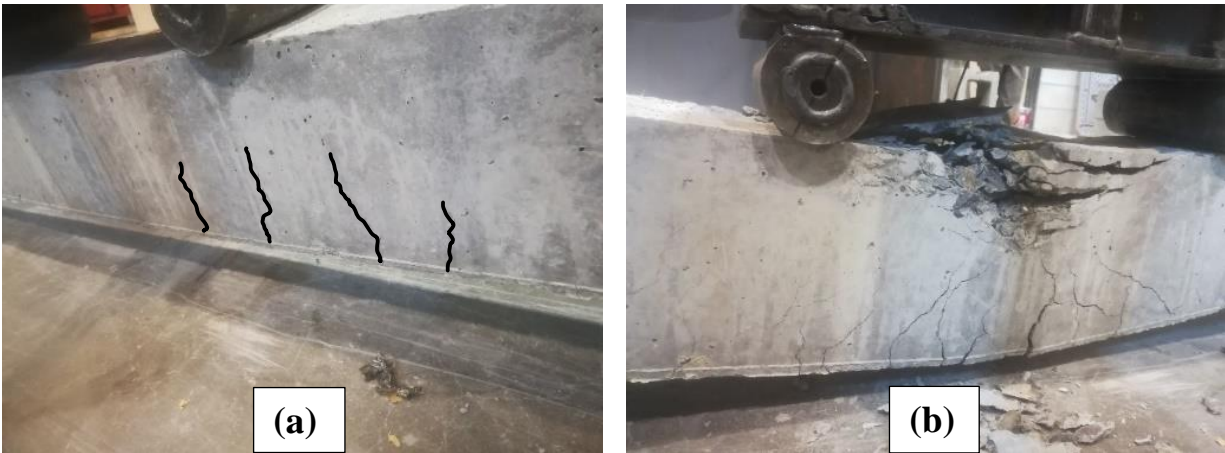
Figure 29. CBRT beam failure; (a) Flexural cracks forming throughout testing, (b) Concrete crushing at end of testing.
