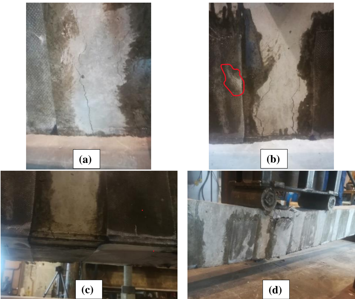
Figure 35. SBLTRT beam failure; (a) Flexural cracks, (b) Delamination of transverse FRP, (c) Debonding of longitudinal FRP and tearing of transverse FRP, (d) Concrete crushing.
