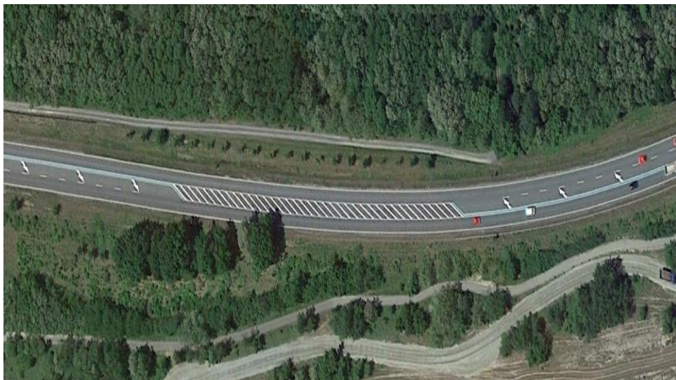
Figure 5. Aerial photo of 2+1 road in Germany (Source: Google Earth)
