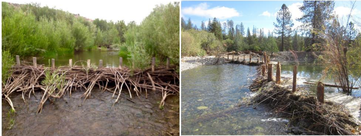
Figure 3. Two examples of Beaver Dam Analogs and Post-Assisted Log Structures installed in Western streams. Branches and organic material are woven between the posts to mimic beaver dams, slowing the flow of water, causing ponding. Sources:
