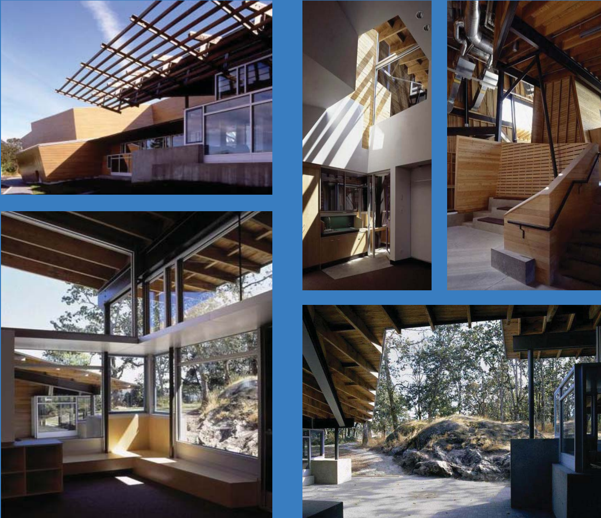
IMAGE SET - FIG. 5.4 - 5.8 The Strawberry Vale Elementary School contains private and public spaces with opulent glazing and seating areas. The use of shadow, materiality, and connectivity with the exterior gives the school a sacred quality. Passive solar features, easily accessible mechanical systems, and other environmental characteristics allow this facility to be very sustainable. http://www.patkau.ca
