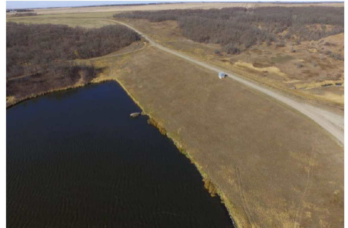
Photo From SE Corner Dam Embankment
