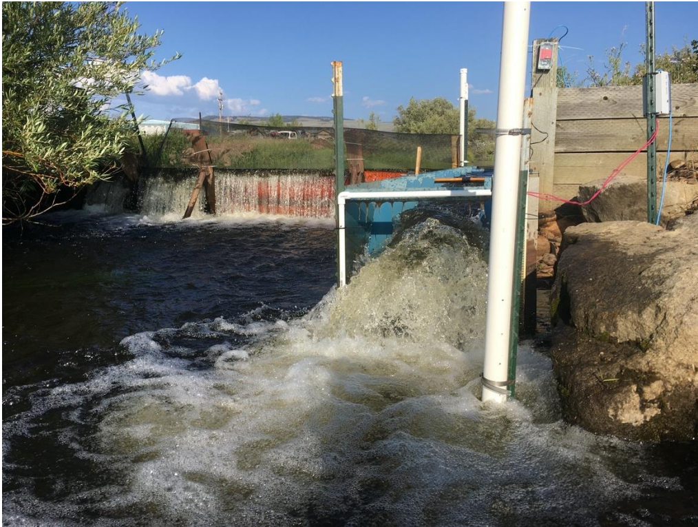
Figure 12: Photo of plunging entrance conditions during Trial 5 on Warm Springs Creek (lower). The deep upstream depth, shallow downstream depth (Table 1), and 0.6% slope resulted in a turbulent entrance plunge that appeared to restrict entrance of Arctic Grayling and limit entrance of suckers during this trial.
