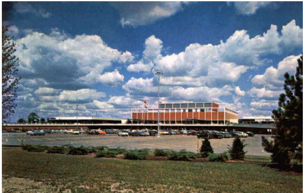
Figure 3-4 Another view of Gruen's mall, this time from the 70s and includ- ing a new design requirement... the sea of parking.
