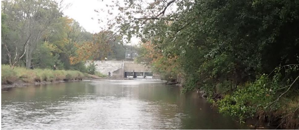
Figure 4. The Fallwell Dam located on the West Branch DuPage River is one of several barriers to fish passage in the Des Plaines River watershed. Others include the Fullersburg Dam on Salt Creek, and the Pilcher Dam on Hickory Creek.
