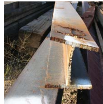
steel structural members
