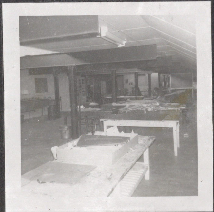
INADEQUATE LIGHTING & INSUFFICIENT WORK SPACE.....
