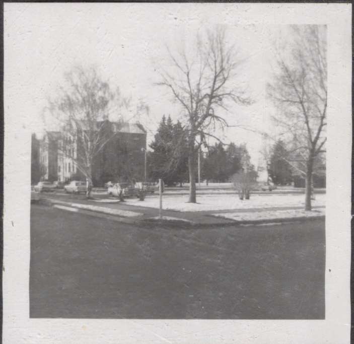
VIEW TOWARD THE SITE FROM SOUTH- EAST.....
