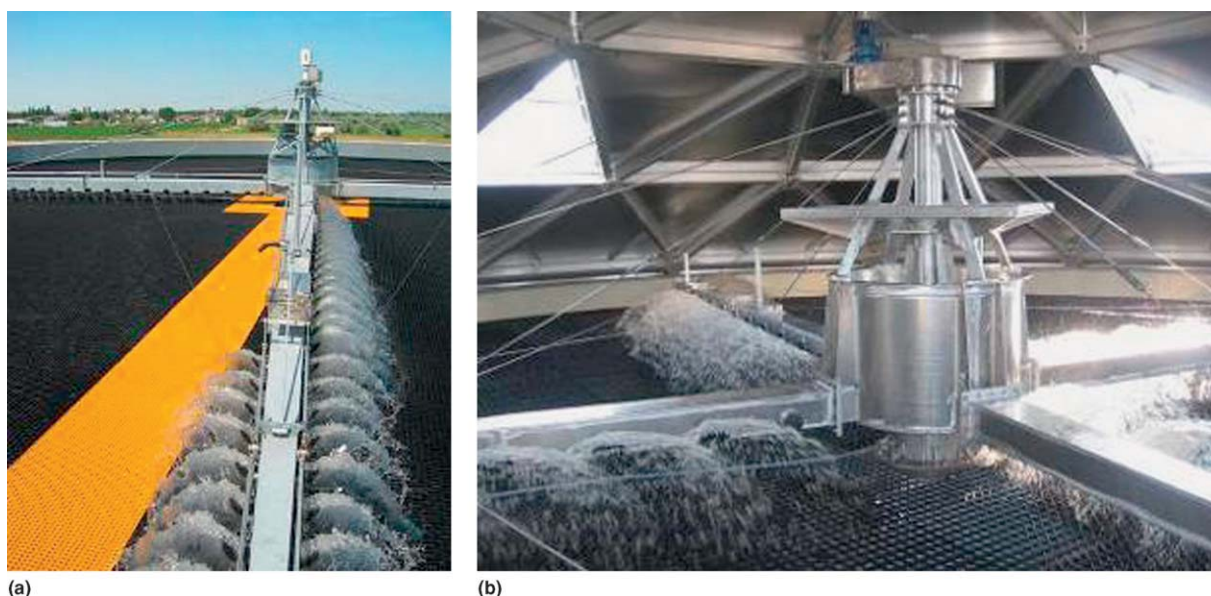
Figure 32 (a) Hydraulically driven rotary distributors use variable frequency drive controlled gates that either open or close distributor orifices which adjust with varying pumped flow rates to maintain a constant preset rotational speed. (b) Electrically driven rotary distributor. Photographs courtesy WesTech, Inc.
