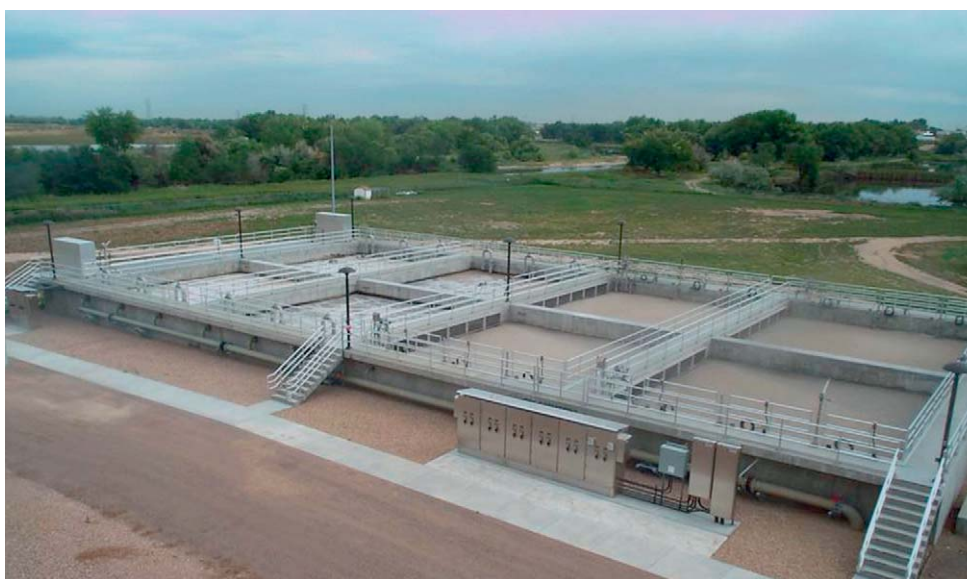
Figure 22 (a) Moving bed biofilm reactor at the Williams-Monaco Wastewater Treatment Plant, Colorado, USA. (b) Schematic representation of the photographed system which illustrates the system consisting of two parallel trains each with four reactors in series.
