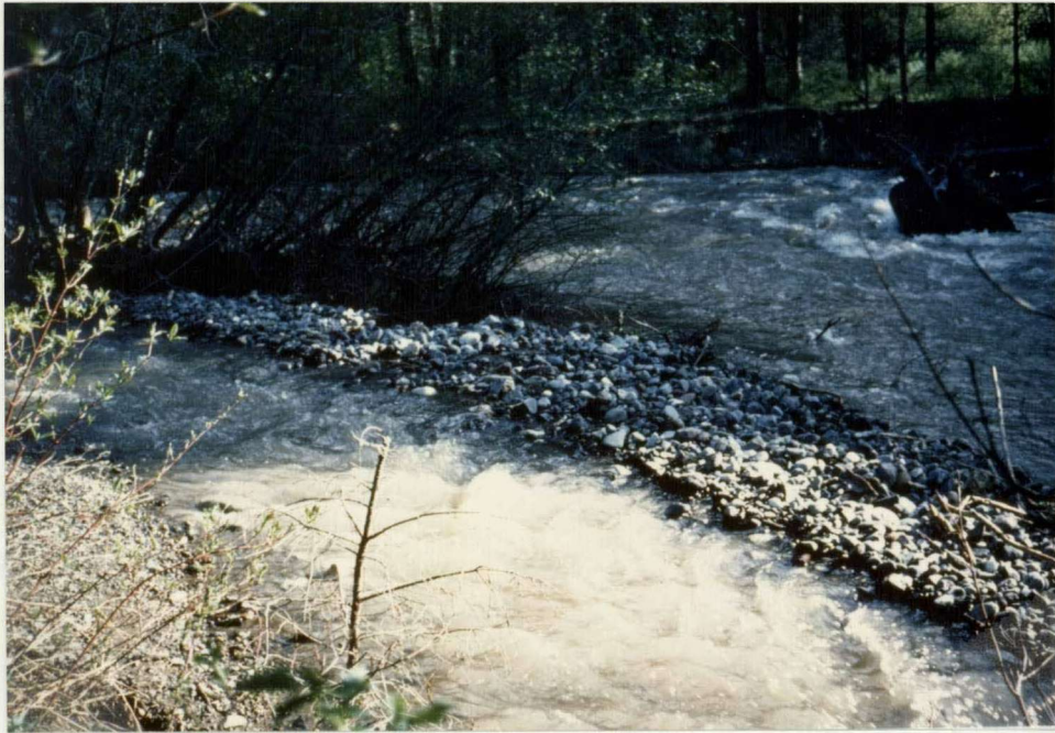
Figure 22. Aggradation of bar along right bank during 1983 bedload event.
