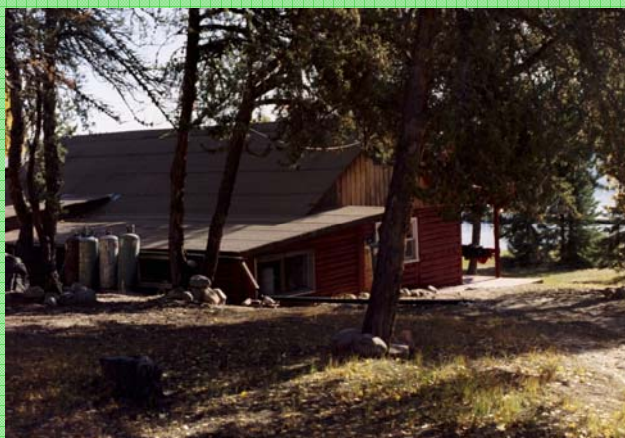
Figure X — Camp Grayling's existing lodge, south.
