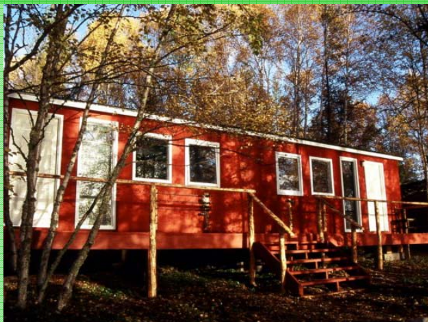
Figure AA — A Camp Grayling existing typical cabin.
