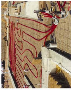
Radiant Floor System
