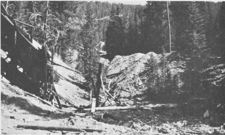
Figure 23. View of the Wasa mine looking east from below the Zimmer Jack adit.
