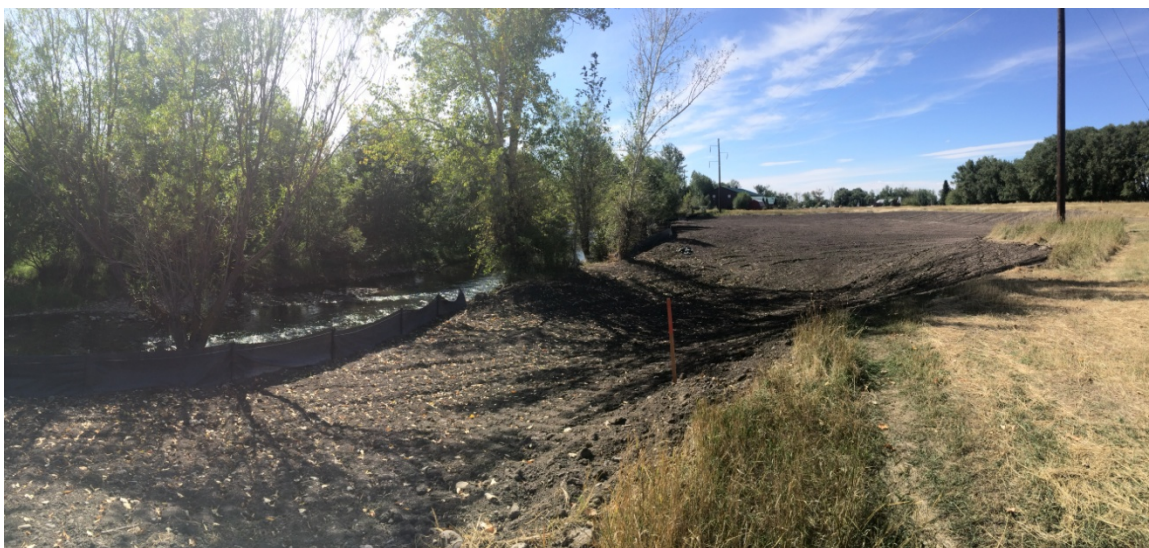
Figure 14. Floodplain excavation along the East Gallatin River, similar to the Bozeman Creek Slough, constructed on the Northern Parcel in September 2015.
