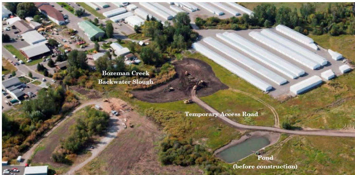
Figure 13. Aerial view of the Bozeman Creek Slough during construction in September 2014 (taken from RESPEC Consulting and Services (2015)).
