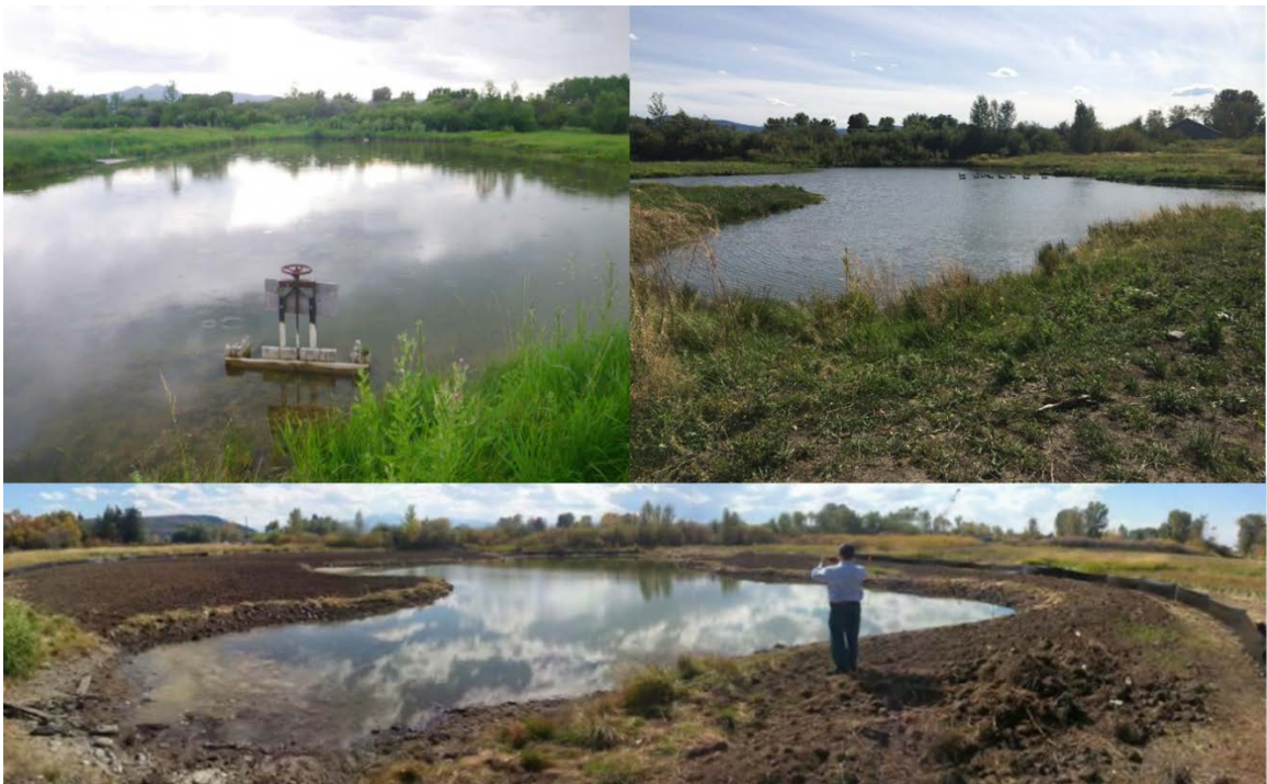
Figure 16. Recontouring the Pond. Top Left: Original pond construction with a sluice gate to drain into the ditch. The pond was contained by tall berms of soil. Top right: Pond one year after construction. Bottom: Pond directly after construction, with lowered bank and no sluice gate (taken from RESPEC Consulting and Services (2015)).
