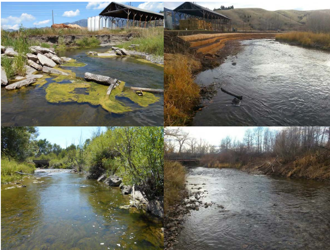
Figure 18. Before (left) and after (right) pictures of the East Gallatin River. Several tons of concrete and metal were removed from the river bed and banks. In the top series, where the river flows past private property, more natural bank stabilization was employed to ensure any resulting creek hydraulics did not undercut the bank (taken from RESPEC Consulting and Services (2015)).
