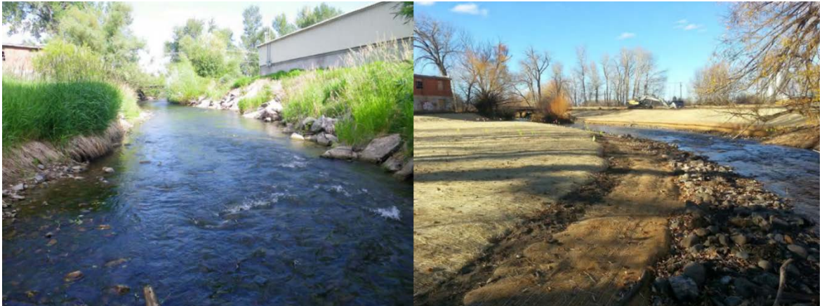
Figure 15. Floodplain excavation along the East Gallatin River on the Triangle Parcel, completed in November 2014. Tall river banks were dug down and back to create a more connected riparian zone (taken from RESPEC Consulting and Services (2015)).
