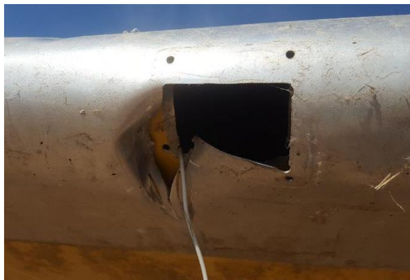
Figure 42. Damage from test 1
