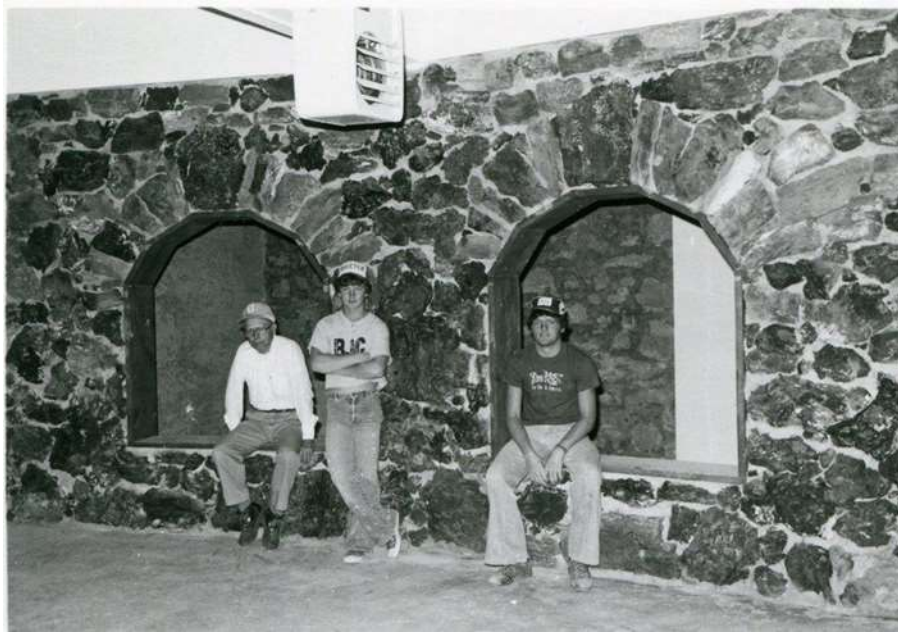
Figure 6. Marshall Lambert and high school students Garth Quade and Norton Walker posing in front of the stone arches they helped construct in the new museum building. Image courtesy Carter County Museum archives.
