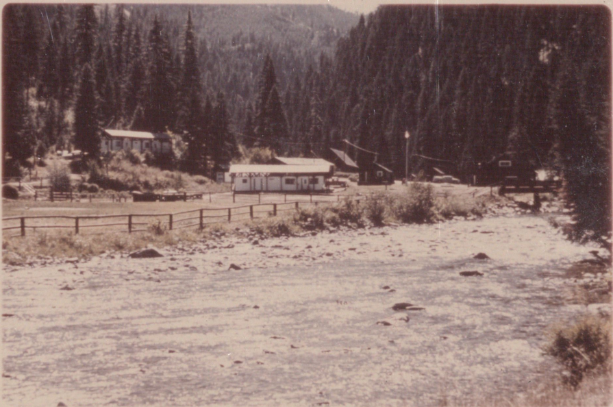
Central Portion of Station
