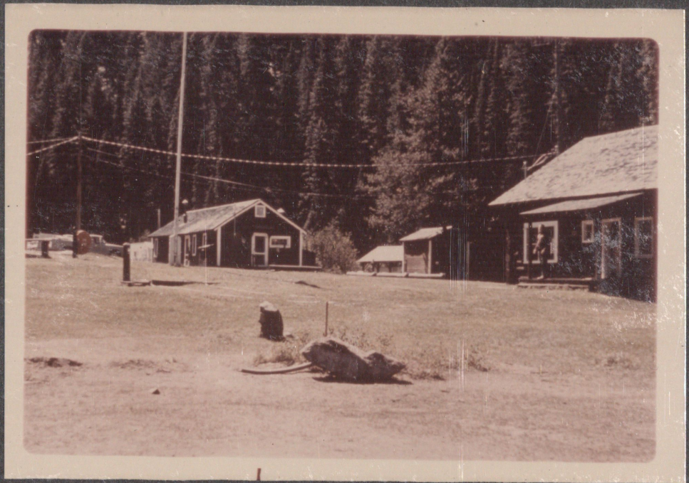
Cook House & Office
