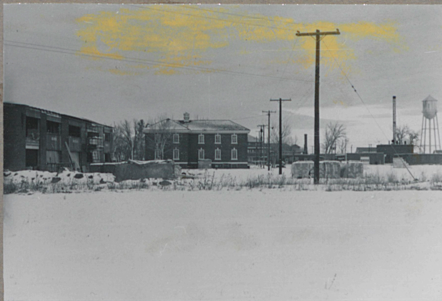
View towards the north
