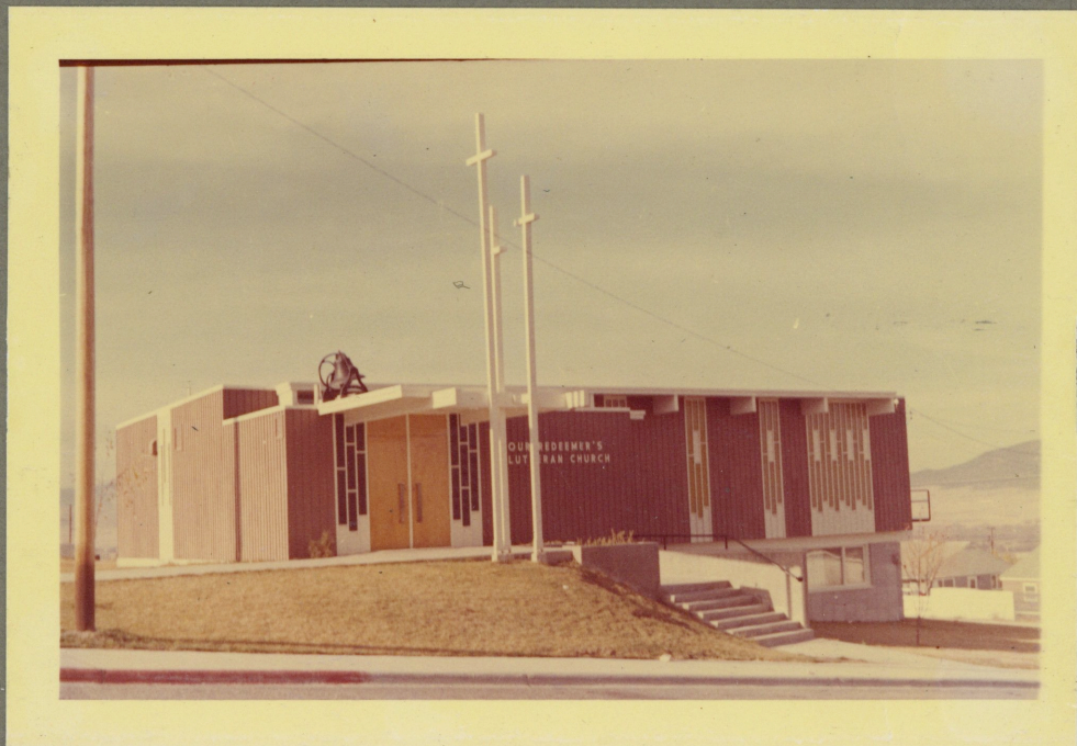
East Side - Main Entrance
