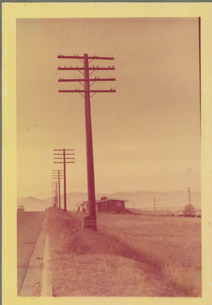
Telephone & Power Poles On Stuart Avenue
