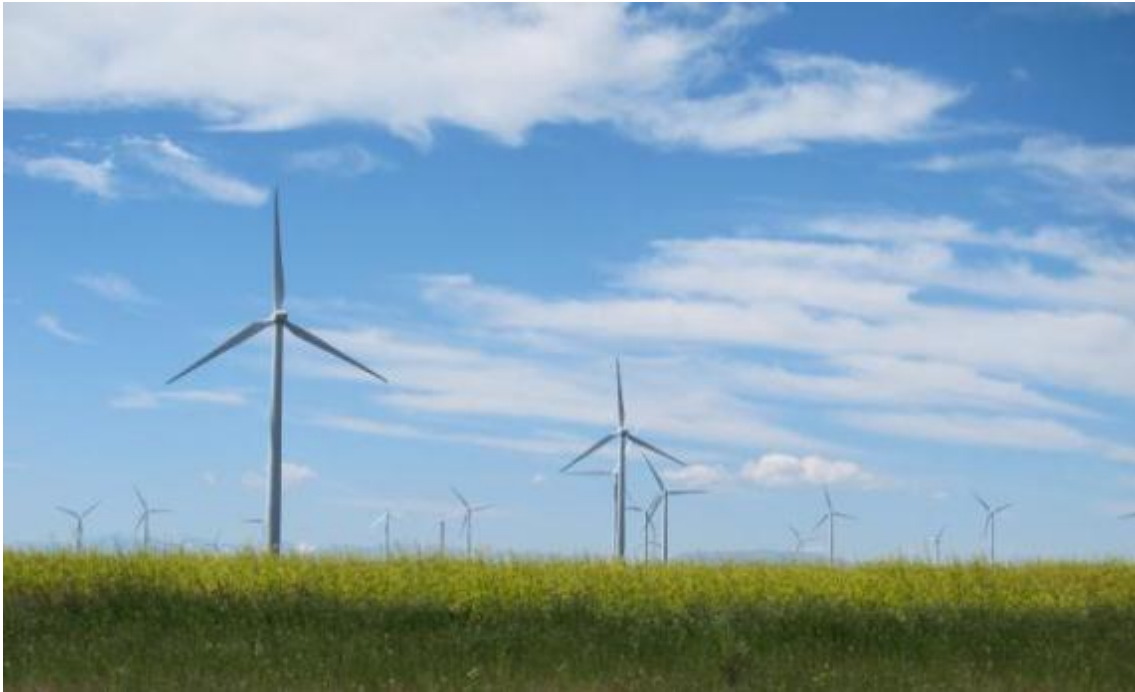
Figure 5. The Judith Gap Wind Farm in Montana
