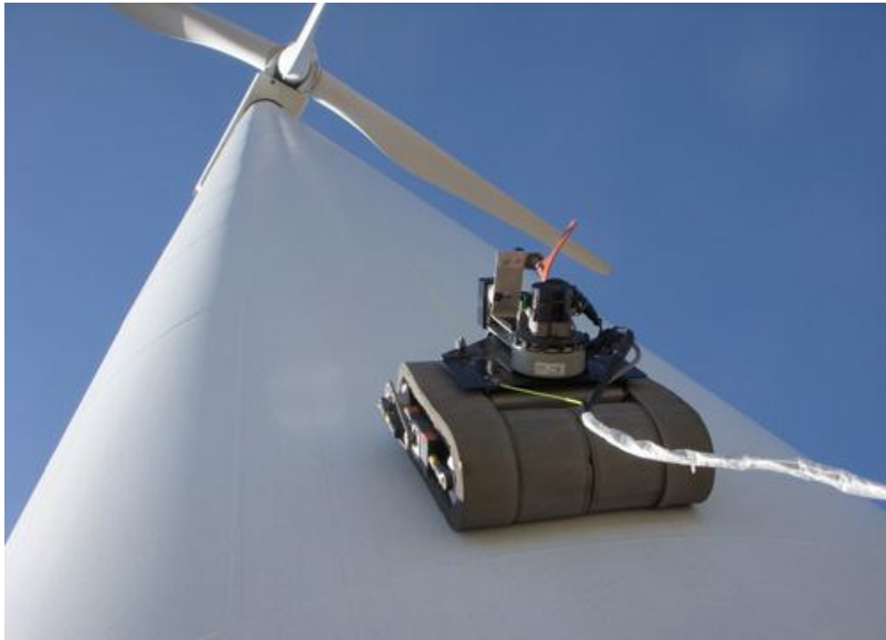
Figure 2. GE's remote-controlled wall climbing robot used to photograph the blades and look for failure points
