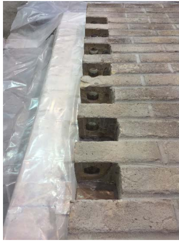
Figure 17: Shear keys present in confined masonry wall
