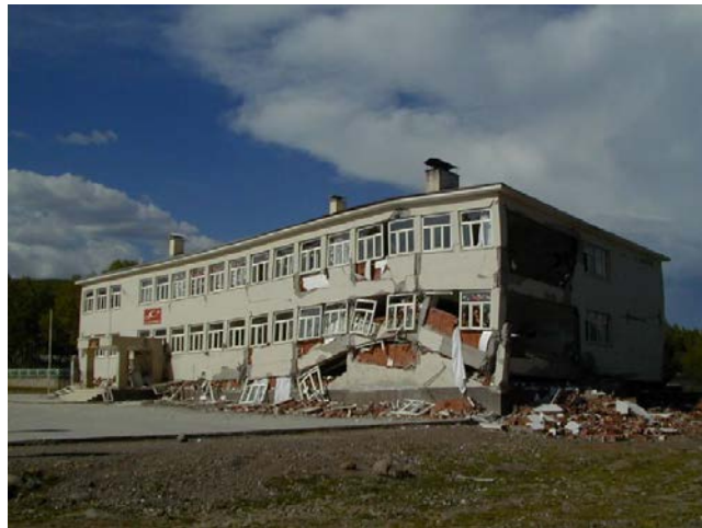
Figure 74: School building in Bingol, Turkey that suffered collapse in the 6.4 Mw earthquake (DataHub 2015)
