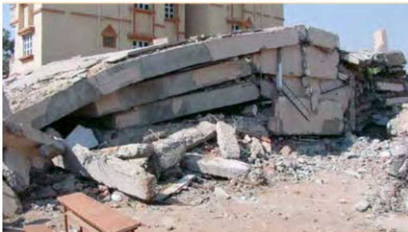
Figure 5: Building collapse due to strong beam-weak column design in 2001 Bhuj, India earthquake (Murty, Brzev et al. 2006)
