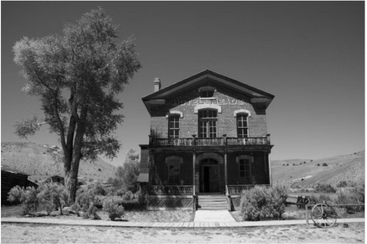
FIGURE 3.4(a). The Meade Hotel at Bannack State Park. The Meade Hotel served many purposes in Bannack during its boom days. Prior to becoming a hotel, it served as Beaverhead County Courthouse. It was one of several structures that underwent restoration under the guidance of Roy Herseth. Source: Image courtesy of William Wyckoff.
