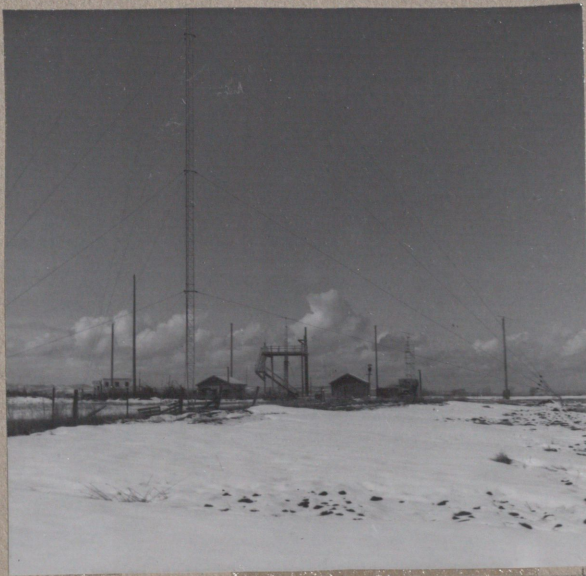
ANTENNAE & LOG CABINS
