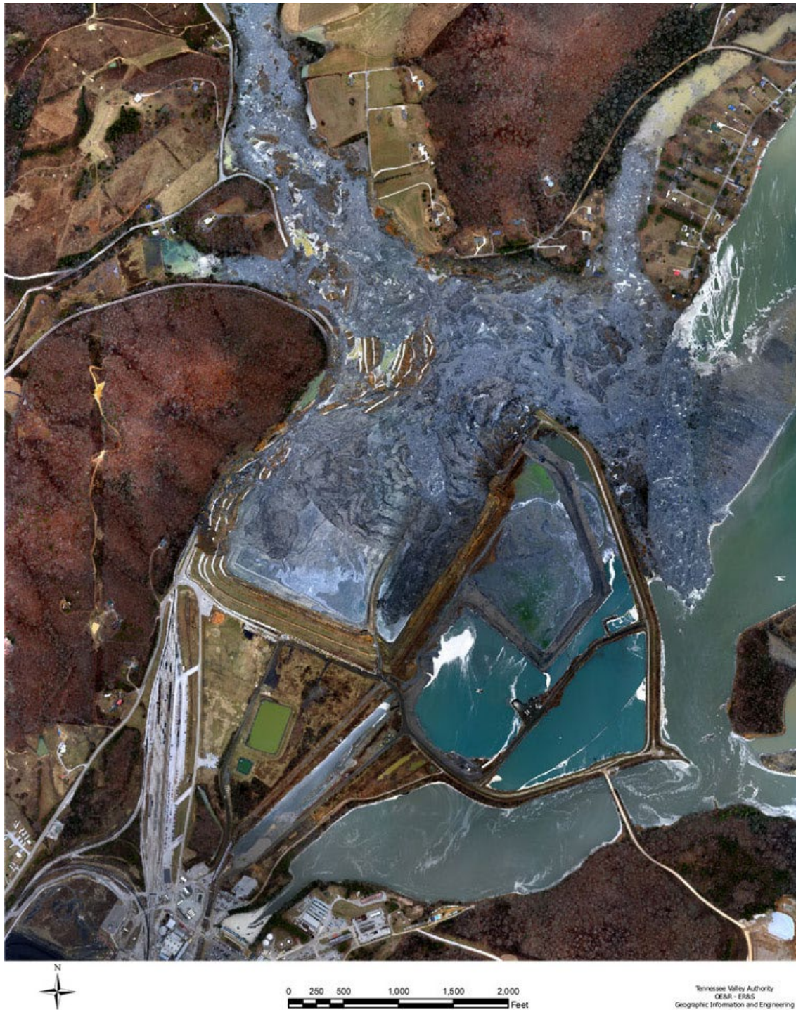
Figure 7: Aerial View of the Coal Ash Spill at the Tennessee Valley Authority's Kingston Power Plant, indicating extent and visible nature of the spill (Sturgis 2014)
