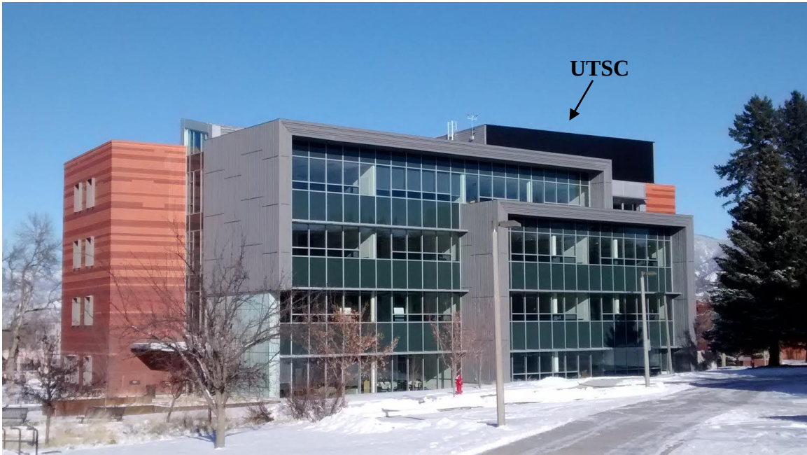
Figure 4: View of the south side of Jabs Hall. UTSC is highlighted in above image.
