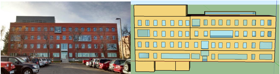
Figure 18: View of Jabs Hall from the north. Left - photograph. Right - energy model.
