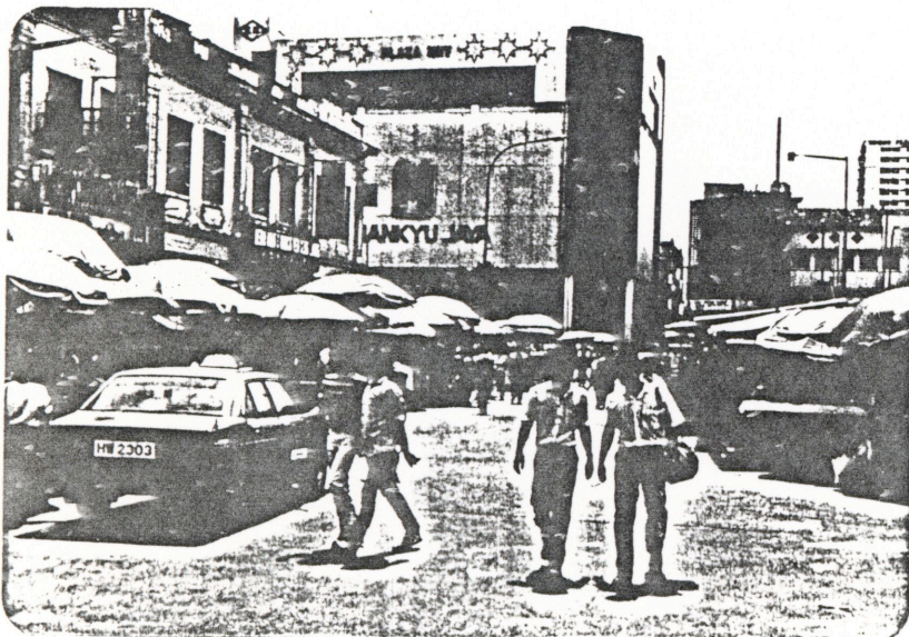
VIEW: TOWARD JLN. TUANKU ABD. RAHMAN FROM THE SITE. (MAIN ENTRANCE TO THE SITE)
