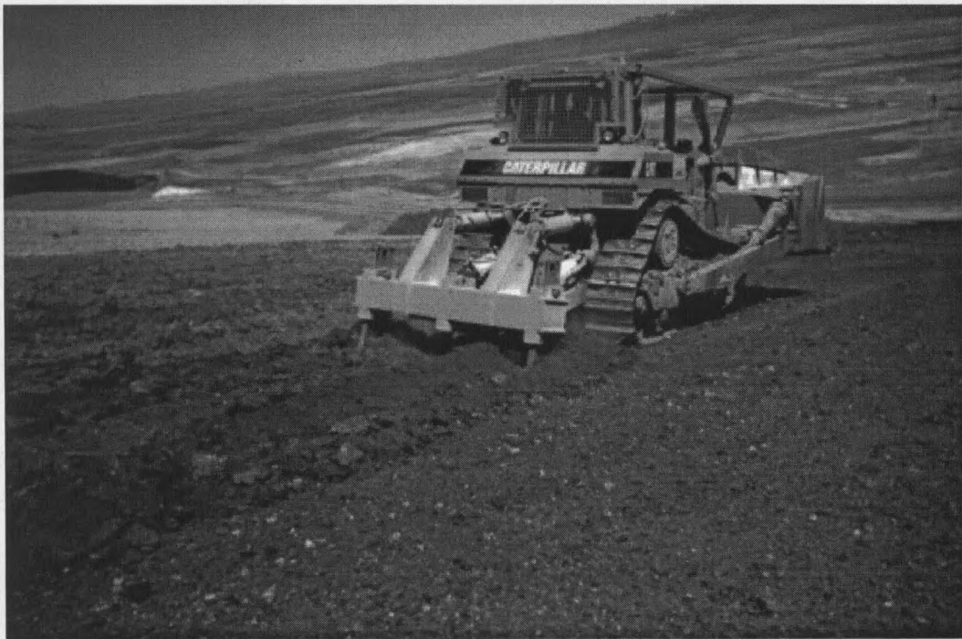
Figure 5. Two ripper shanks ripping to 2 feet with a D8N dozer.
