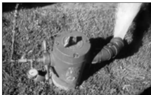
Unidirectional flushing may remove deposit-associated coliforms from distribution systems.
