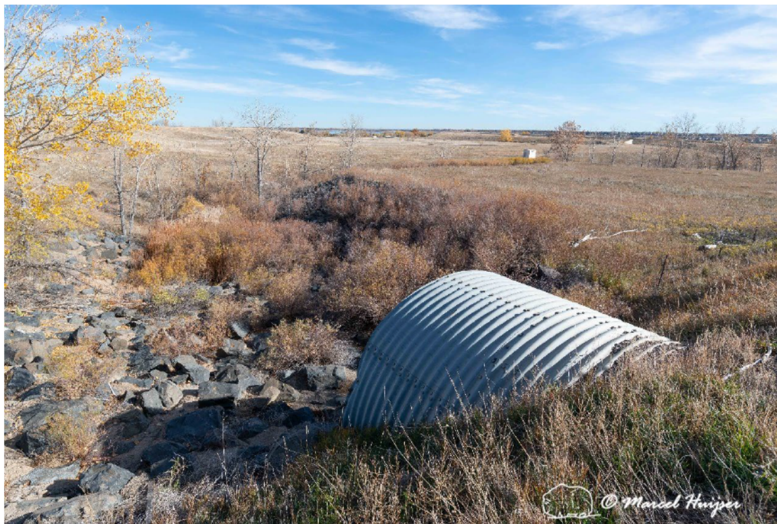
Figure 32: Riprap at outflow, South Woman Creek (Indiana St., 2.25 mile south of junction with Hwy 128), east side, outflow.
