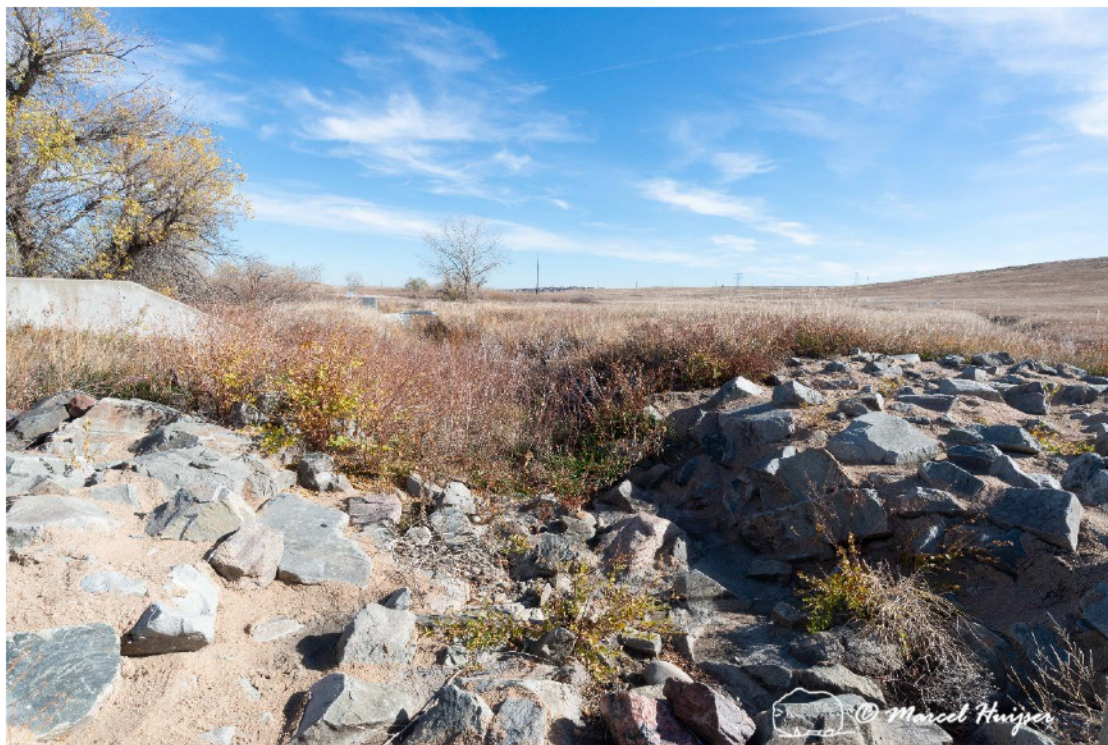
Figure 29: Riprap at outflow, Walnut Creek (Indiana St., 0.62 mile south of junction with Hwy 128), east side, outflow.
