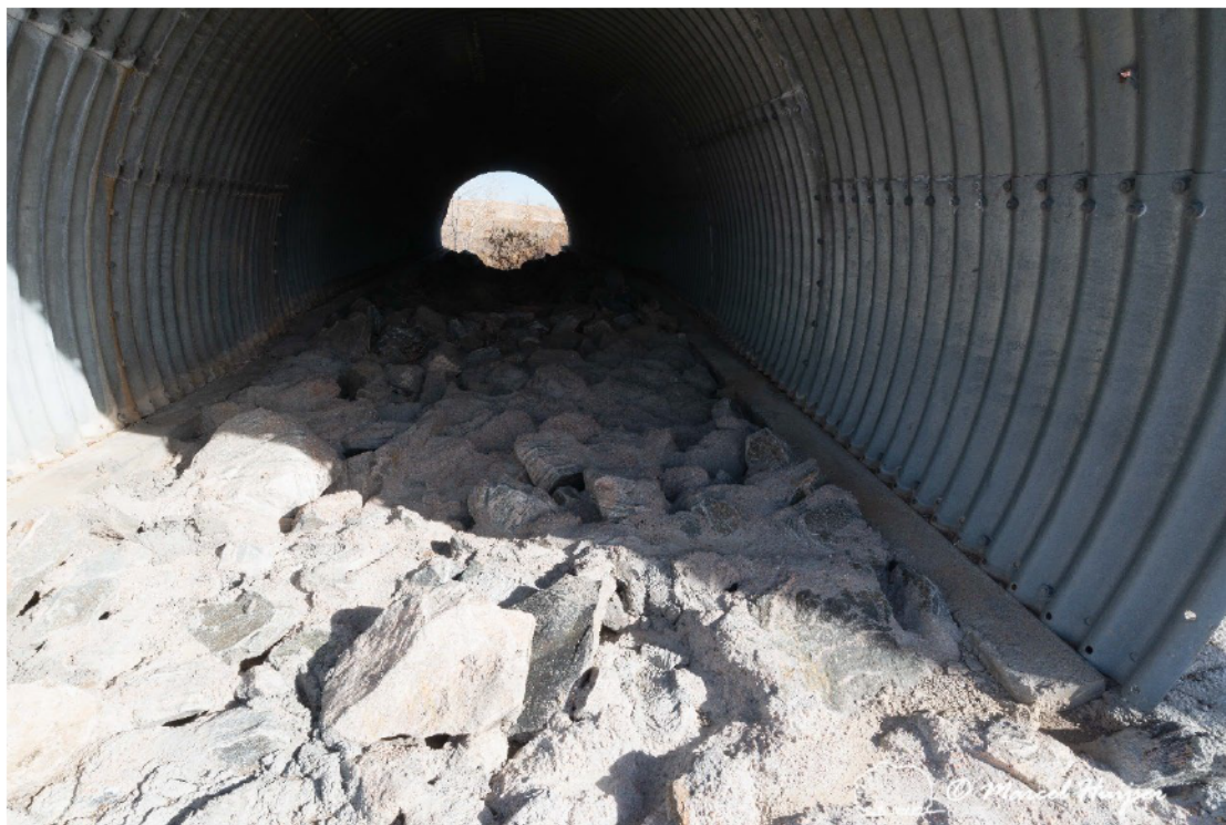
Figure 31: Riprap inside culvert, South Woman Creek (Indiana St., 2.25 mile south of junction with Hwy 128), west side, inflow.
