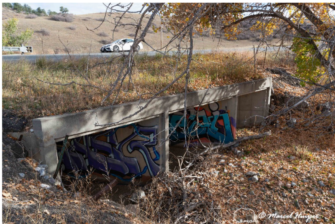
Figure 20: Divided box culvert, Coal Creek (Hwy 93, mile reference post 10.95), west side, inflow.
