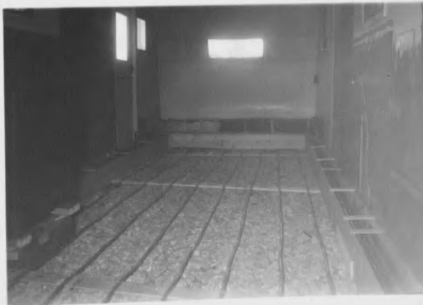
Figure 4 North End Bottom Panel
