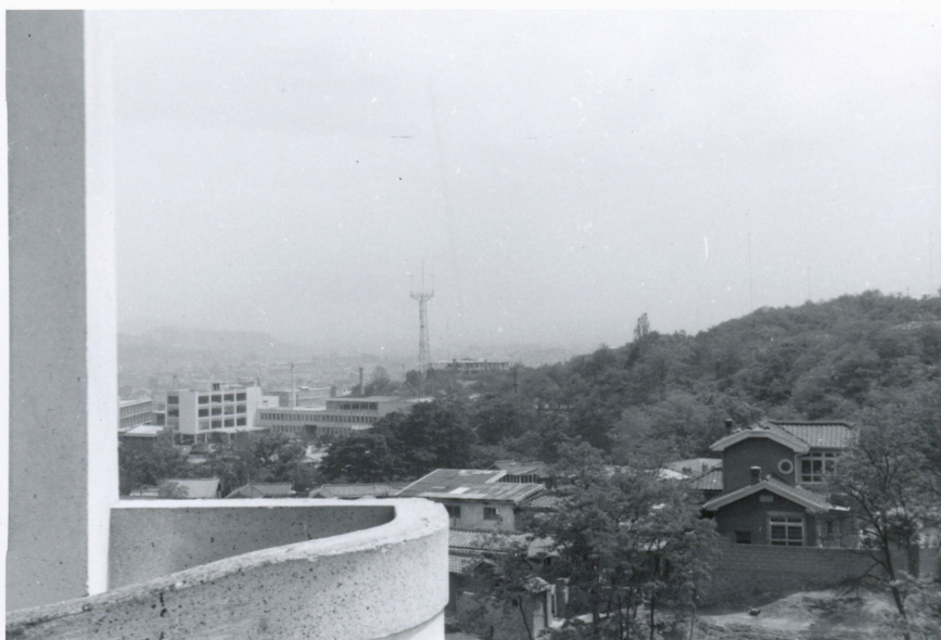
VIEW TOWARD NORTH-EAST
