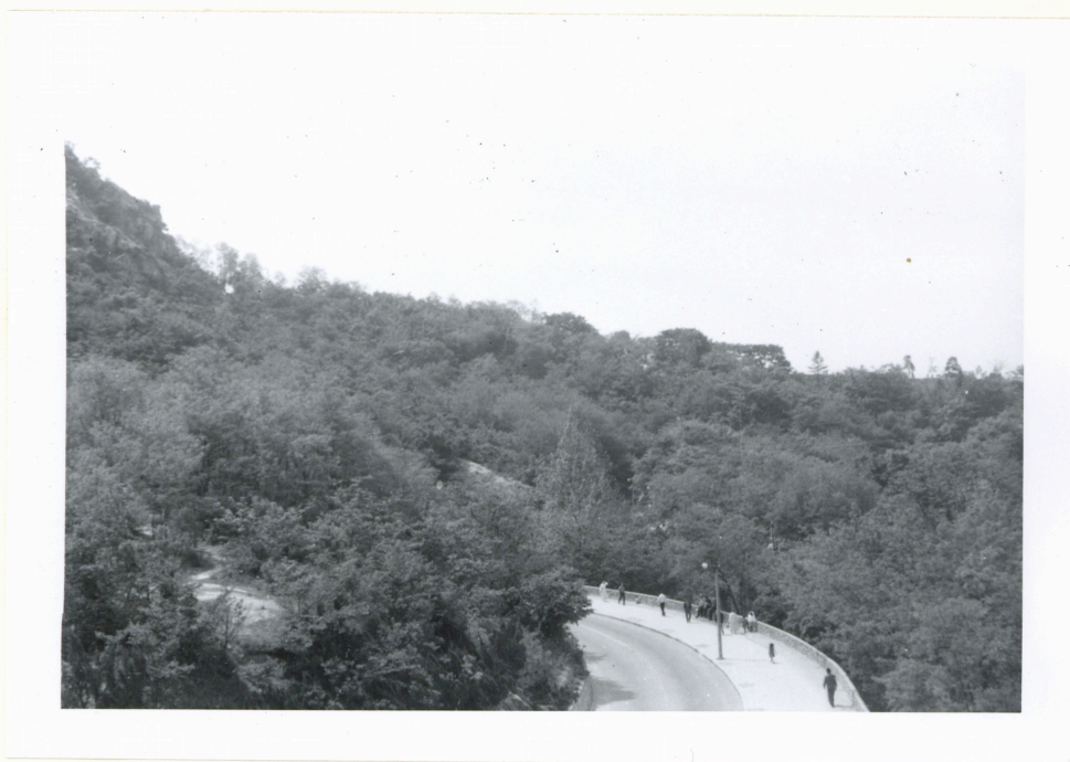
VIEW TOWARD SOUTH-WEST
