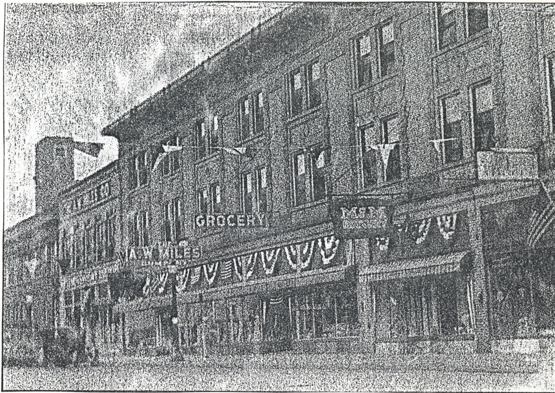
A.W. Miles Building and the Miles Block. (c. 1920)
