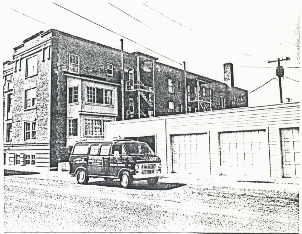
East elevation of unfinished brick.
