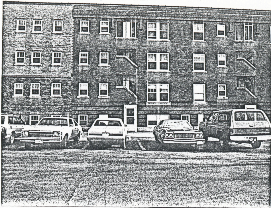
North elevation showing rear stairways.
