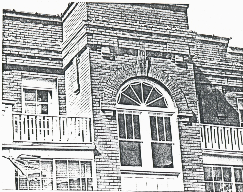
Detail of balconies and stairwell window.
