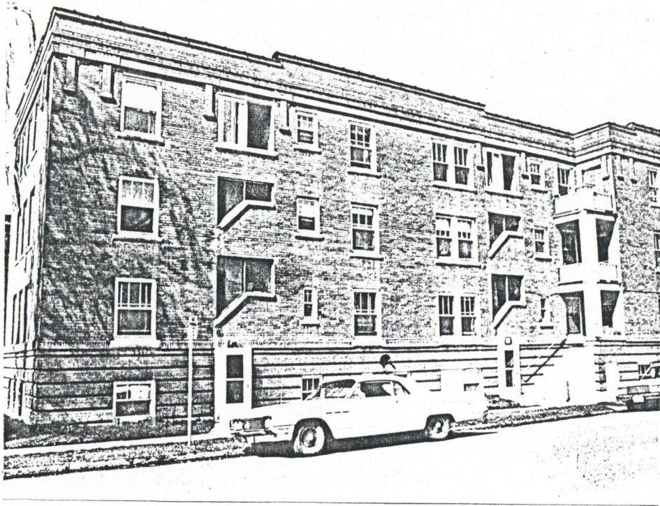
South elevation showing rear stairways.
