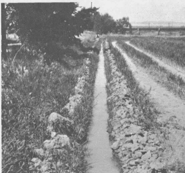
Figure 10. Surface water sampling site for quality analyses in the surface drain approximately 300-feet from the plots.
