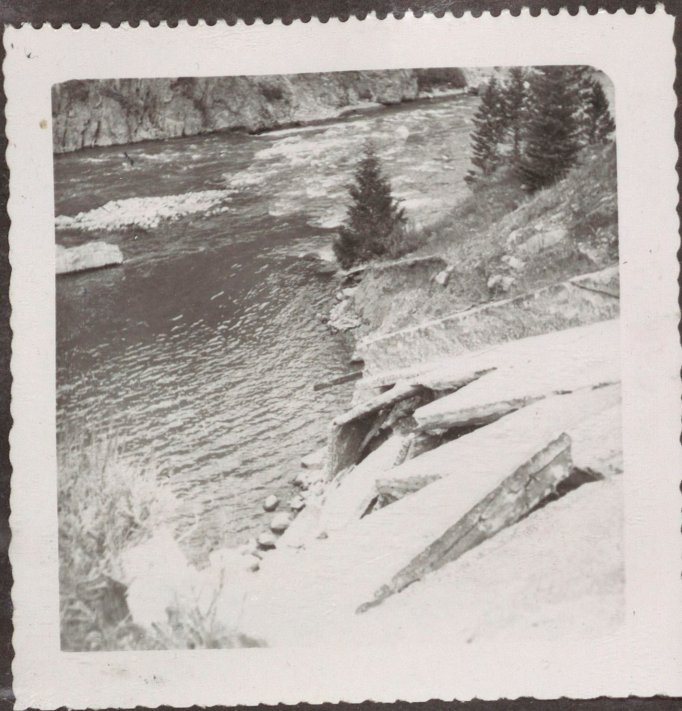
FIGURE 17 SPILLWAY AT HEBGEN DAM
