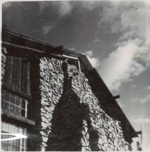
FIGURE 4 CHIMNEY IN WEST YELLOWSTONE
