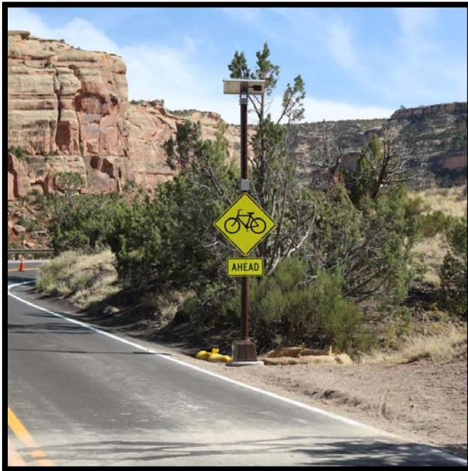
Figure 2. Site 1 after the installation of the Dynamic Bicycle Detection and Warning System facing North.
