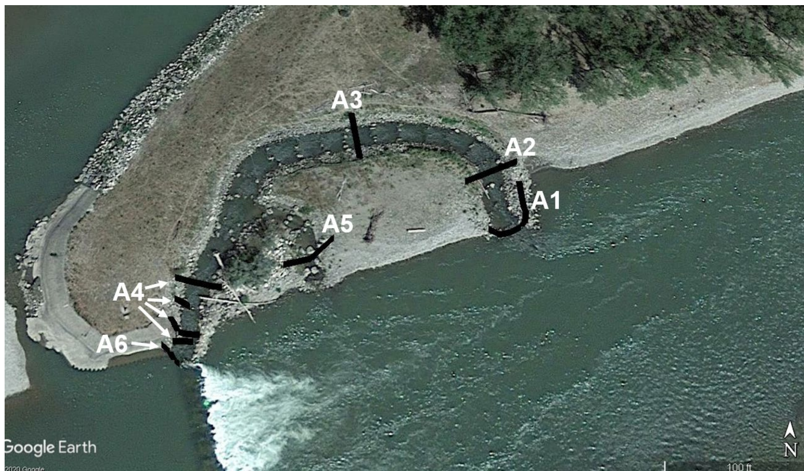
Figure 2. Locations of stationary PIT antennas used to monitor the movement of tagged fish during the evaluation of the nature-like fishway at Huntley Diversion Dam, Yellowstone River, Montana, from April 23, 2019, through December 31, 2020.
