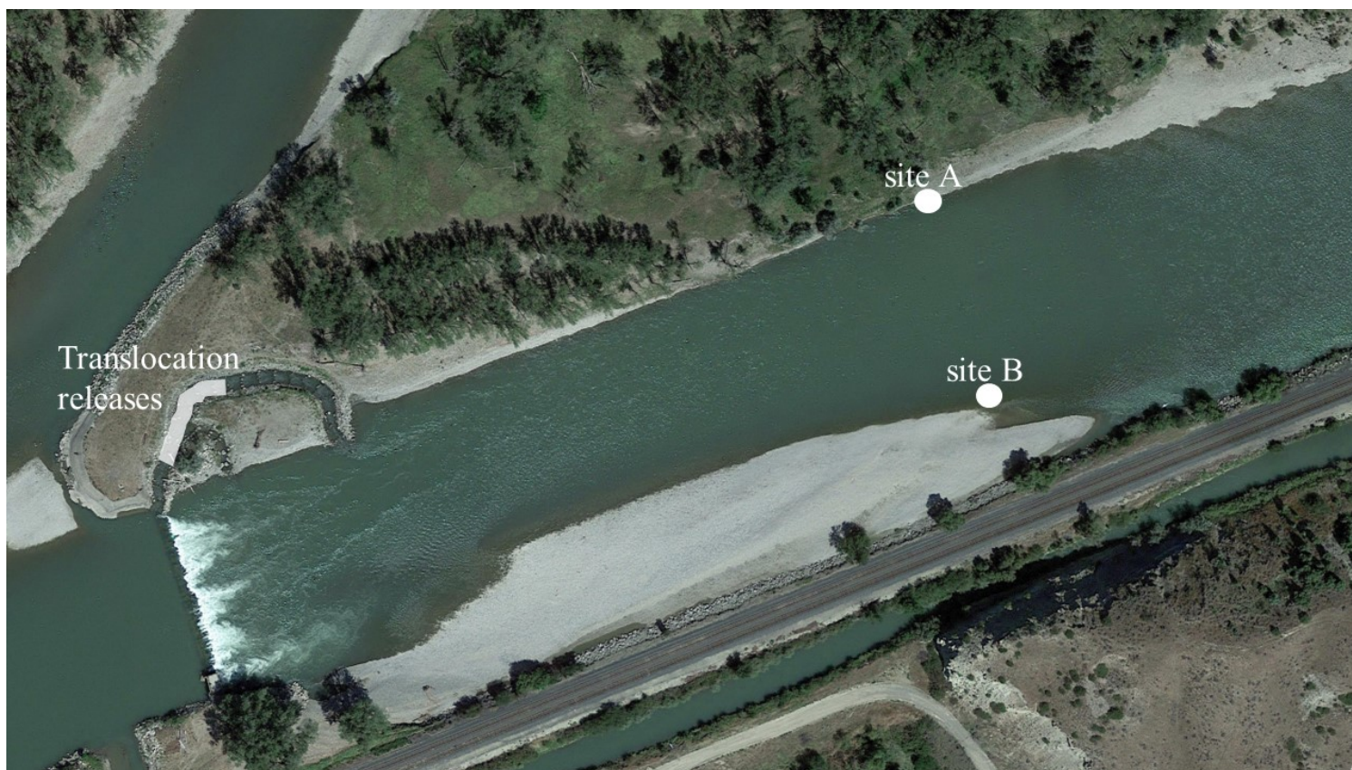
Figure 1. Release sites of PIT-tagged fish in the general group (see Methods for definition) and translocated Saugers used in the evaluation of the nature-like fishway at Huntley Diversion Dam, Yellowstone River, Montana, in 2019 and 2020.
