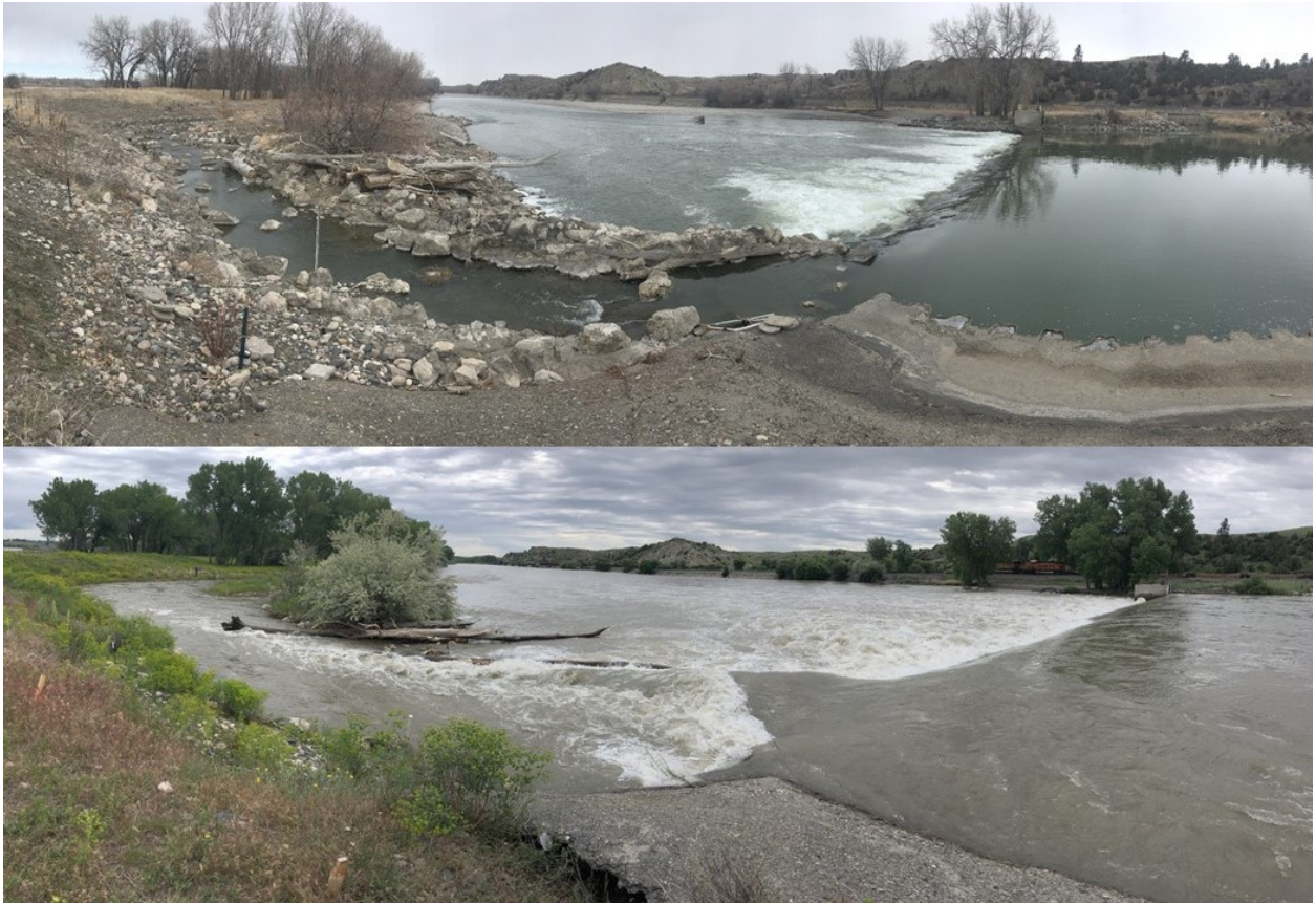
Figure 15. Photos of the exit of the nature-like fishway at Huntley Diversion Dam, Montana, at low ( 78 \text{ m}^3/\text{s} ; 2,750 \text{ ft}^3/\text{s} ; upper panel) and high ( 1,002 \text{ m}^3/\text{s} ; 35,400 \text{ ft}^3/\text{s} ; lower panel) discharges of the Yellowstone River. A rock wall forming the downstream side of the fishway exit and a reinforced concrete shelf are visible at low discharges, whereas both become entirely submerged at high discharges. Note the water plunging off of the concrete shelf and into the fishway at high discharges, as well as the standing wave formed where water flows over the rock wall. These problematic hydraulic conditions at high discharges delay successful fish at the exit and probably prevent others from passing.
