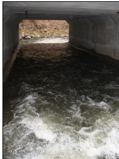
Interior of Culvert 1, looking downstream, flow rate estimated at 37.5 cfs.
