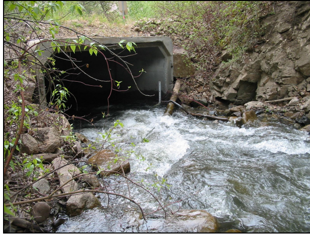
Inlet region of Culvert 1, looking downstream, flow rate estimated at 37.5 cfs.
