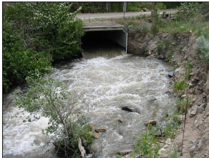
Outlet region of Culvert 1, looking upstream, flow rate estimated at 120 cfs.
