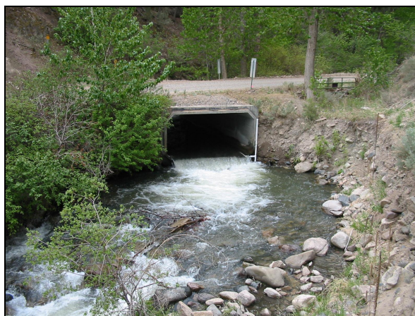
Outlet region of Culvert 1, looking upstream, flow rate estimated at 37.5 cfs.
