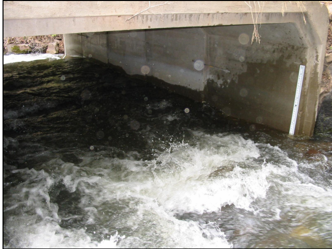
Inlet region of Culvert 2, looking downstream.
