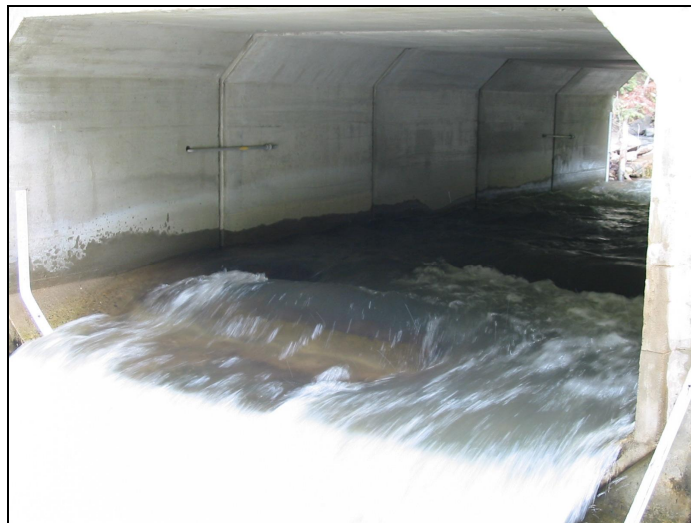
Outlet region of Culvert 2, looking upstream.
