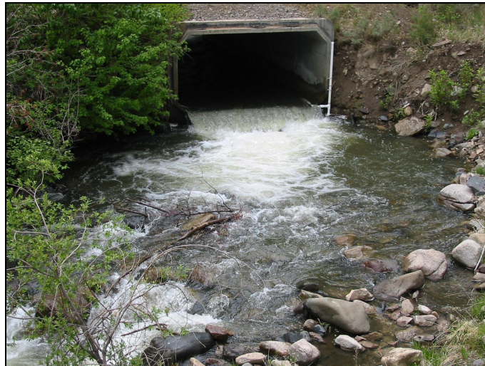
Outlet region of Culvert 1, looking upstream, flow rate estimated at 28 cfs.
