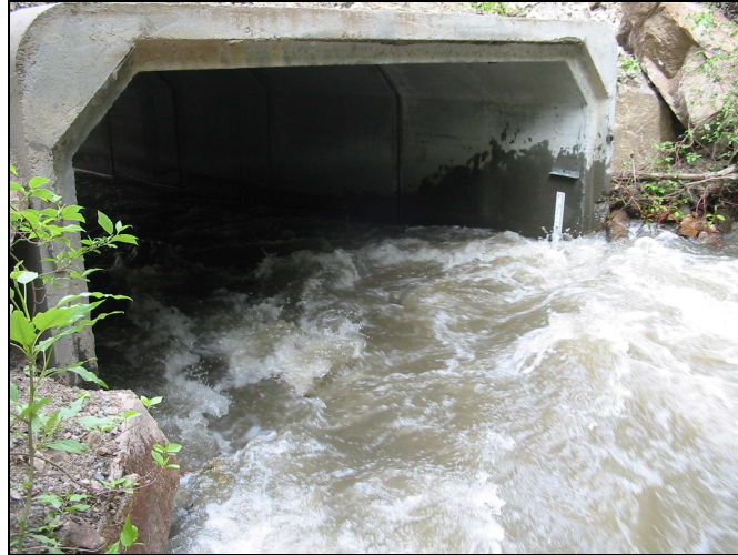
Inlet region of Culvert 1, looking downstream, flow rate estimated at 120 cfs.
