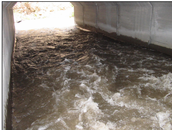
Interior of Culvert 1, looking downstream, flow rate estimated at 120 cfs.
