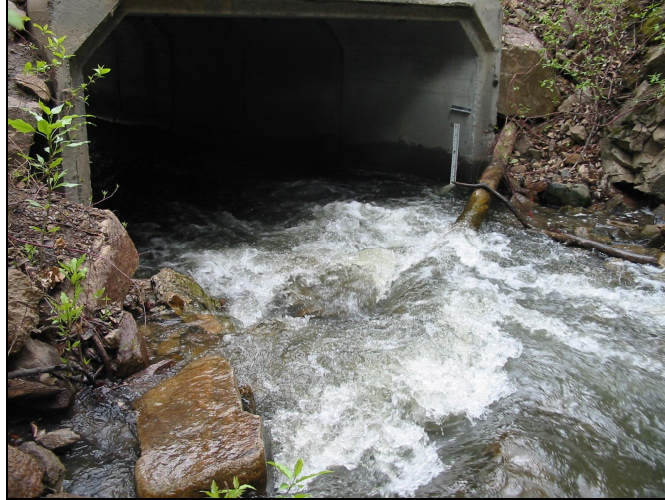
Inlet region of Culvert 1, looking downstream, flow rate estimated at 28 cfs.
