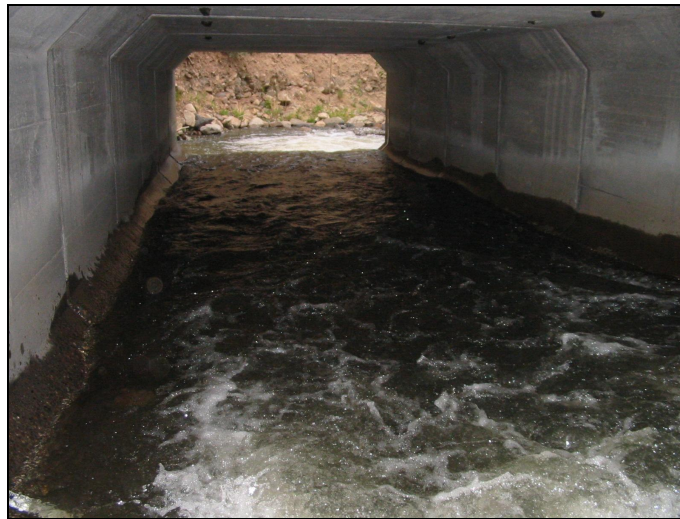
Interior of Culvert 1, looking downstream, flow rate estimated at 28 cfs.
