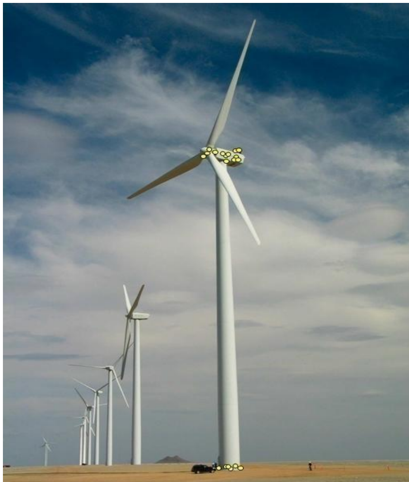
Figure 3. Location of current sensors monitoring turbine health and efficiency [8]
