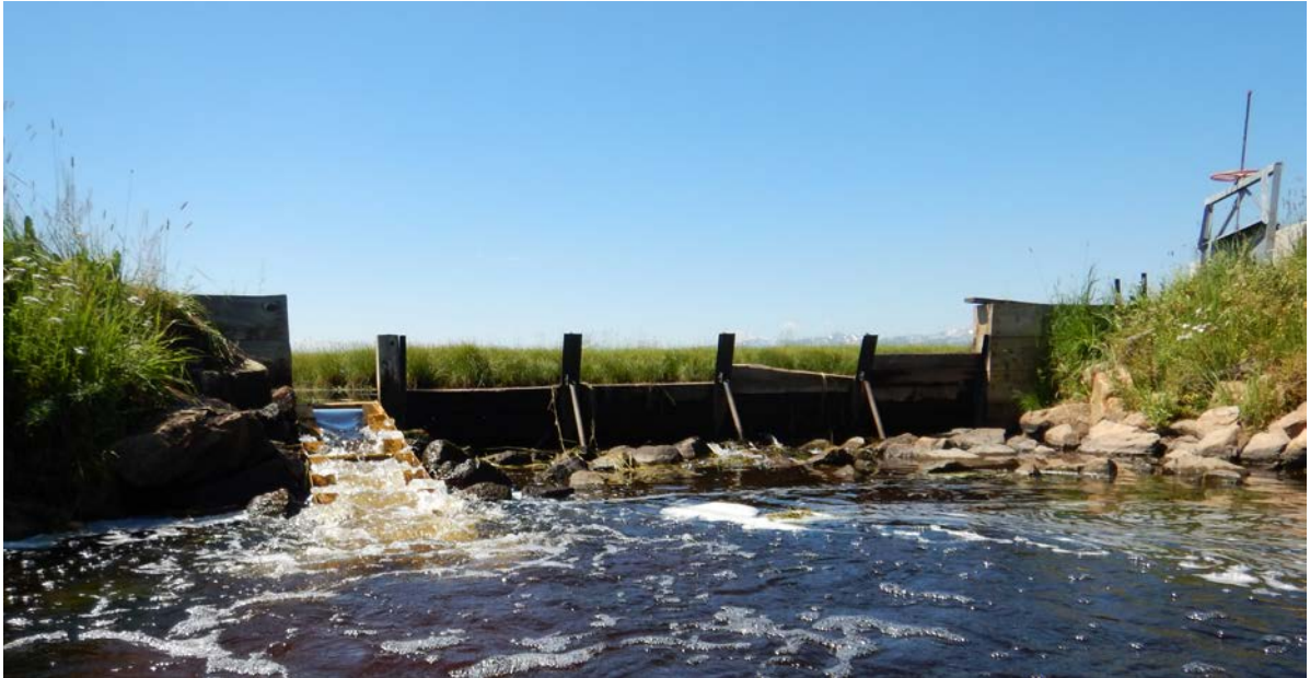
Figure 3.2. Photo of a pin-and-plank irrigation diversion retrofitted with a Denil Fishway, on Swamp Creek in the Big Hole Valley. Note that the diversion is being operated with planks inserted and the fishway is the only route up for moving fish. On the right, the top of a sluice gate which controls the discharge that flows into the irrigation ditch can be seen.
